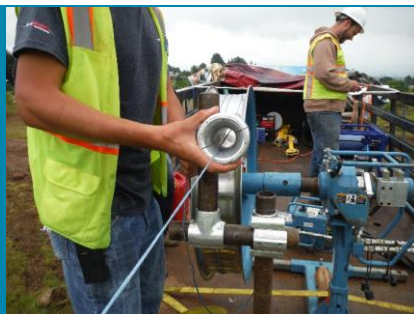
Capstan winch pulling string/cable
