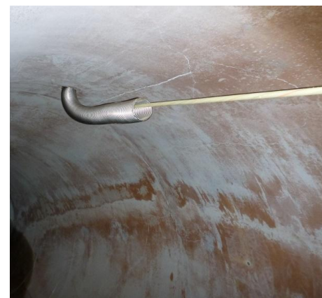
Cable protection into pipe
