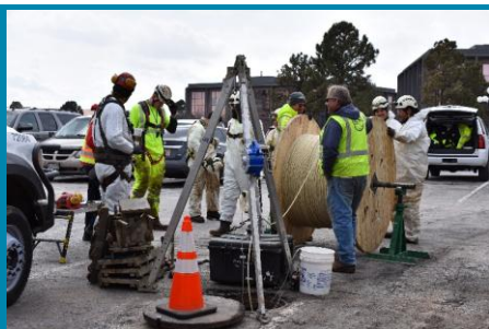
Cable installation staging
