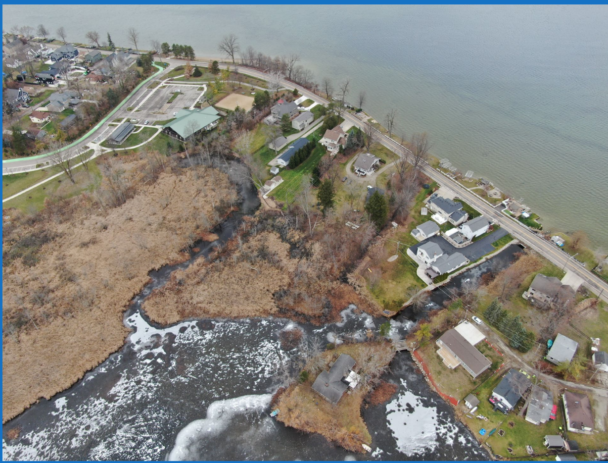
Overhead of "canals"
