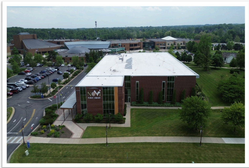
Photograph 2: Typical view of building exterior elevation
