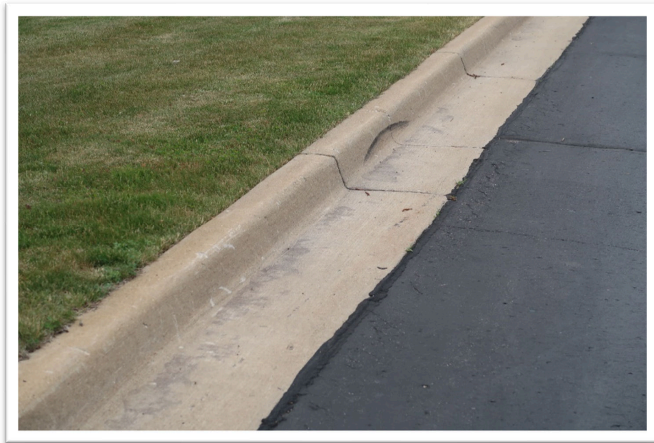
Photograph 29: Typical view of concrete curb
