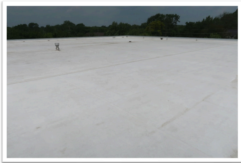
Photograph 5: Typical view of TPO membrane roof cover
