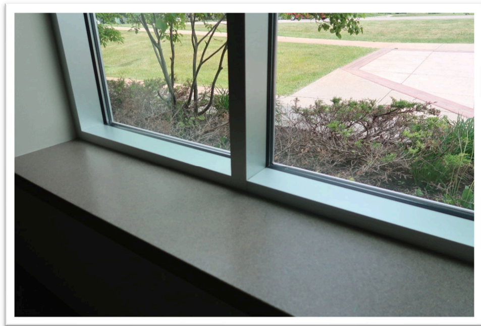
Photograph 9: Typical view of window
