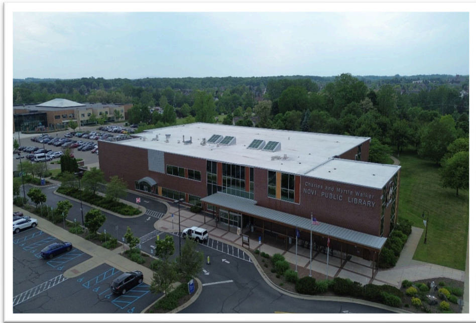
Photograph 1: Typical view of building exterior elevation
