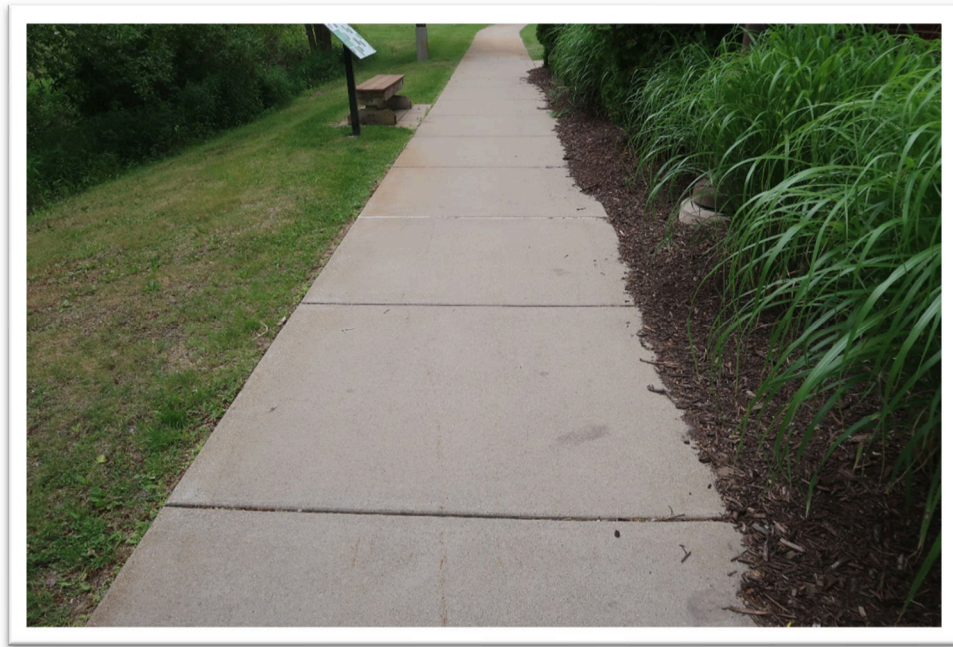
Photograph 25: Typical view of concrete sidewalk
