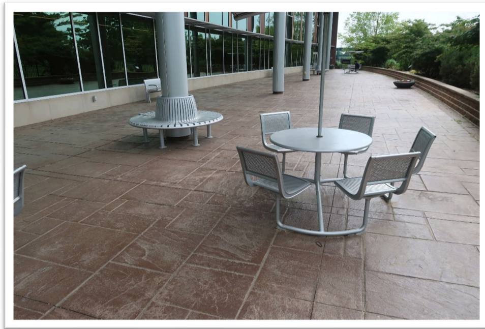
Photograph 27: Typical view of stamped concrete patio area
