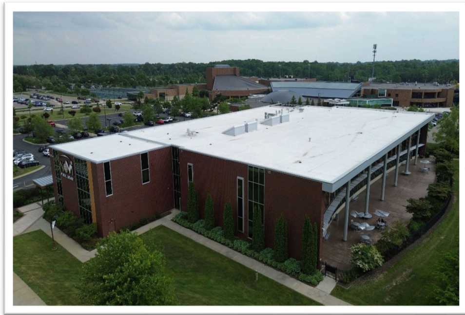
Photograph 3: Typical view of building exterior elevation
