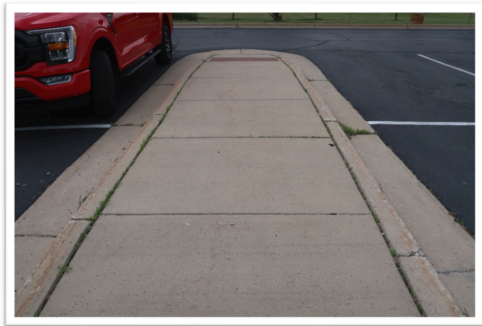
Photograph 26: Typical view of concrete sidewalk
