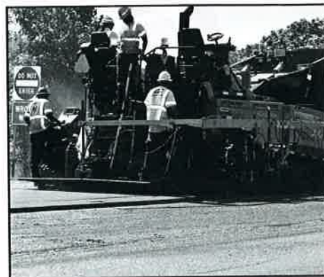
A paving contractor completing an RCOC Preservation Overlay.
