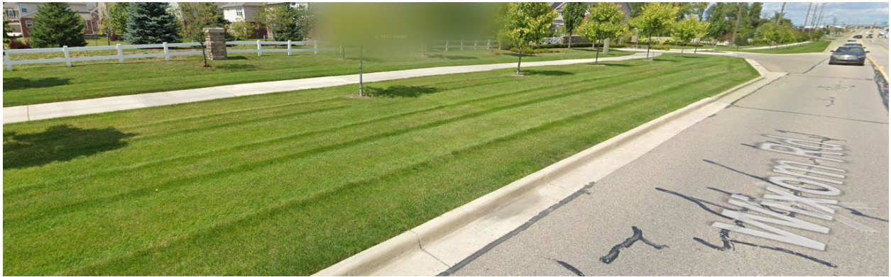
Pic 2 : Before- construction work. Sod Along the Wixom Road
