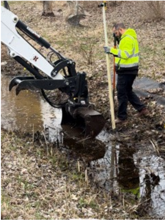
Cleaning a ditch full of sediment
