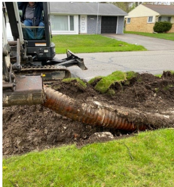
Removing and replacing culverts between ditches
