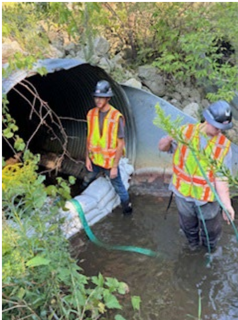
Inspecting high water volume culverts before making structural repairs
