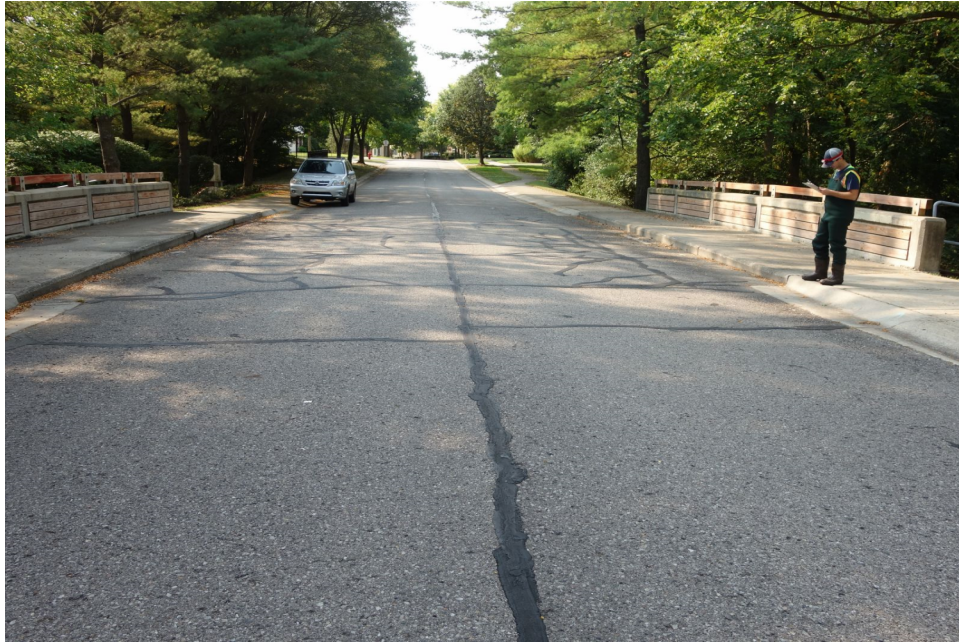
North Approach Looking South
