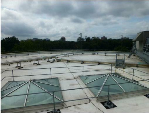
Rooftop at Bldg XXXX
