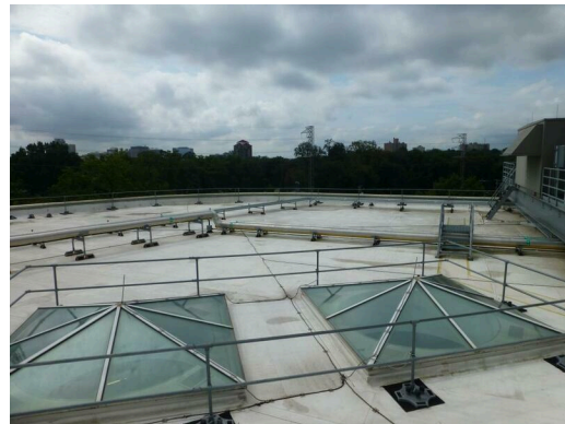
Rooftop at Bldg 1
