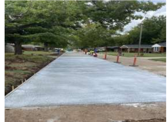
Caddell Lane (Urban Concrete)
