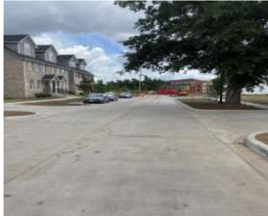
McCullough Street (Urban Reconstruction)
