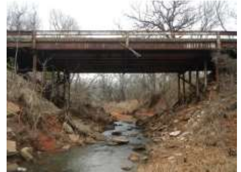
Bridge on 60 th Avenue
