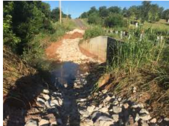
Bridge Maintenance on Cedar Lane
