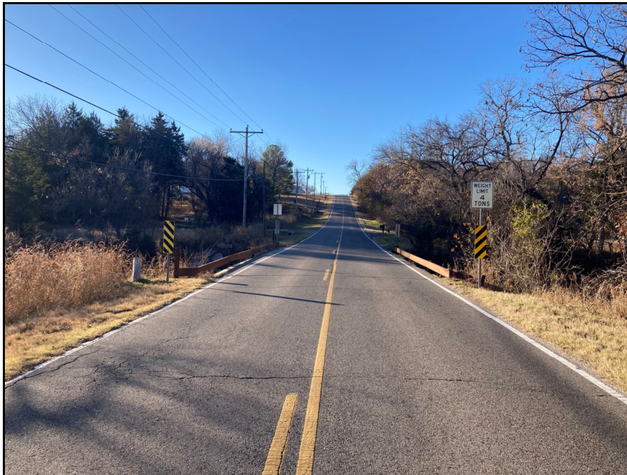
Figure 6 – Load Posting Sign Prior to Bridge Closing
