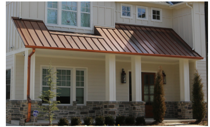
Standing seam metal roof
