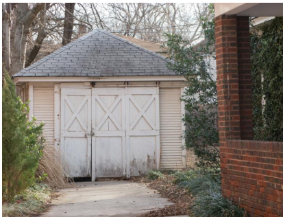
A pyramidal roof was common on single car garages built in the 1920s.
