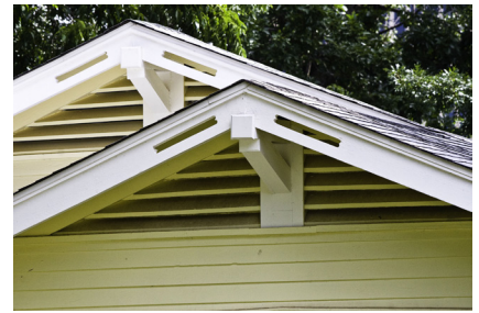
Attic ventilation is accomplished through the use of decorative wooden louvers in a roof gable.
