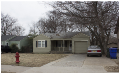
Asbestos shingle siding.
