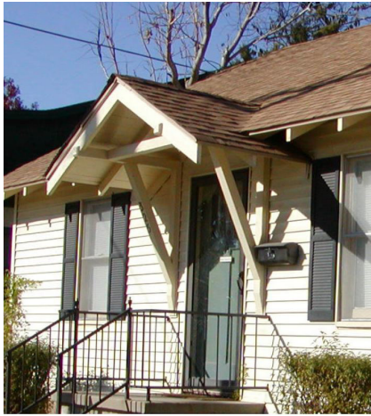
A gablet supported by wood braces provides a decorative covered entrance on this National-style structure in the Miller District.
