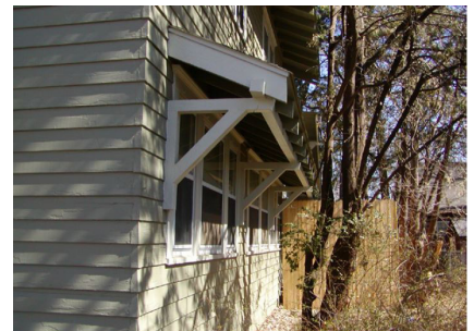
Knee braces support this shed roof over several pairs of windows.
