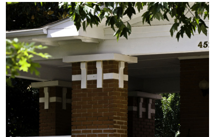
These brick columns on a Craftsman structure also include cast concrete capitals and details.
