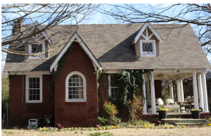
Composition shingle roofing
