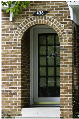
An arched, recessed entryway is characteristic of Tudor Revival structures.
