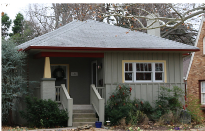
Board-and-Batten siding
