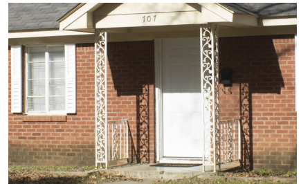
Fabricated metal column
