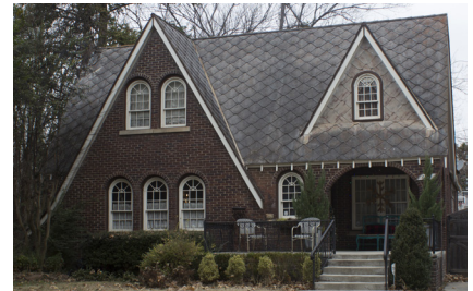
Pressed metal shingle roofing
