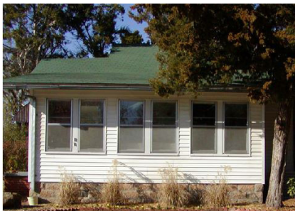
Original window placement often maximizes passive solar as in this south-facing elevation with three pairs of windows.
