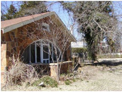
This bungalow has a full-width porch with stone cladding and an unusual elliptical opening.
