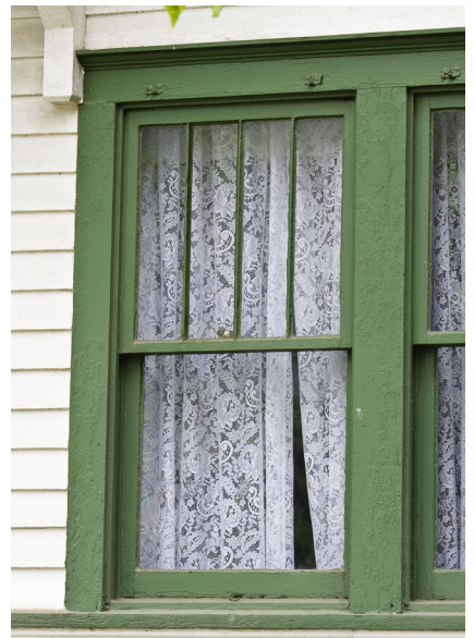
Four-over-one vertical pane configurations are characteristic of Bungalow architecture.
