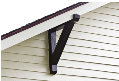
Wood brackets, sometimes known as knee braces, are common decorative support elements on bungalows.
