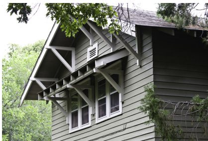
A shed roof supported by brackets provides shade, decorative detail, and support on a Craftsman structure.
