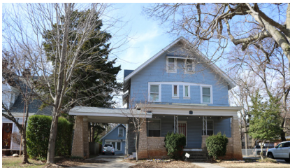
Cut stone piers and columns.
