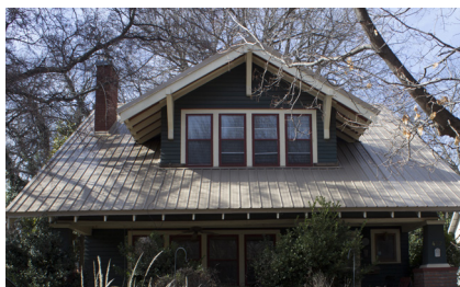
R-panel metal roofing
