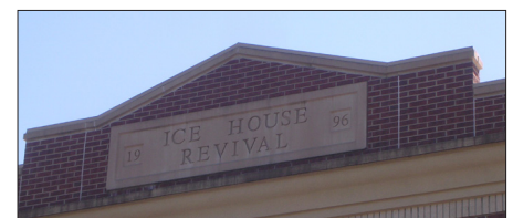
Masonry parapet sign
