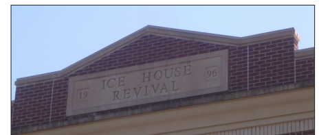
Masonry parapet sign
