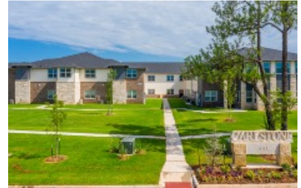
Carlstone Built: 2020 Vacancy: 2.3% Unit Mix: 74 1-Bed, 14 2-Bed Avg Asking Rent: $2,503, $3.26 PSF
