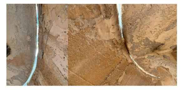
The outboard end of the launder (especially the first 7-8 inches from the bottom of the trough are rusted and deteriorated. The same is true for the lauder support angles (especially the areas where the trough sits on the bracket.)
