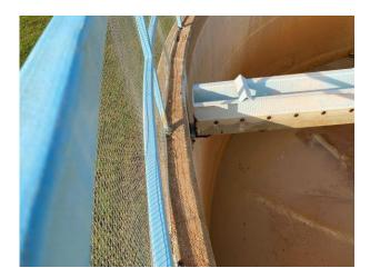
There is rusting in many places, especially at weld points. These have not started to leak, but will sometime in the future.
