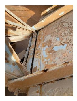
Steel pitting in scraper truss
