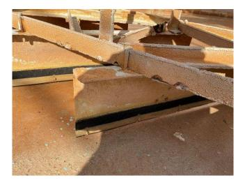
Turnbuckles severely corroded
