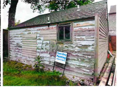
REAR (EAST) – ACCESSORY STRUCTURE
