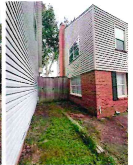
NORTHWEST – PRIMARY STRUCTURE
