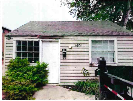
FRONT (WEST) – ACCESSORY STRUCTURE
