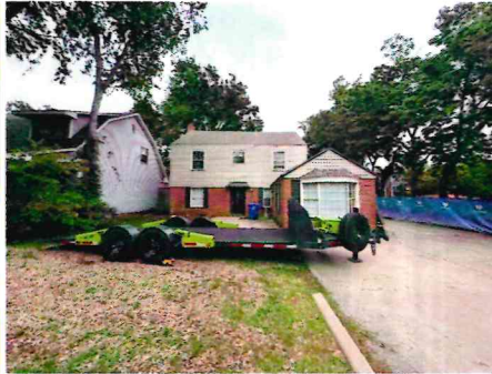
FRONT – PRIMARY STRUCTURE
