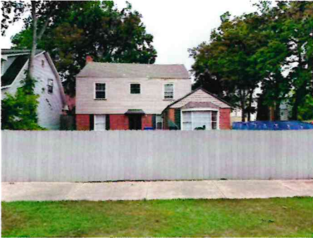
FRONT – PRIMARY STRUCTURE
