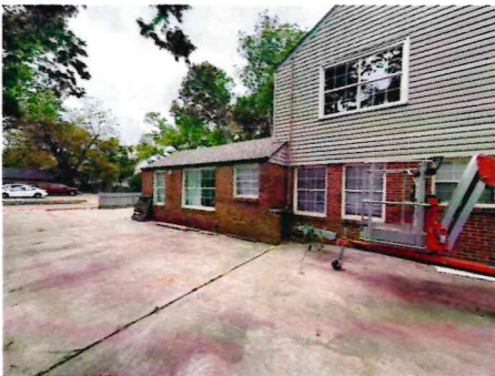
SOUTH – PRIMARY STRUCTURE
