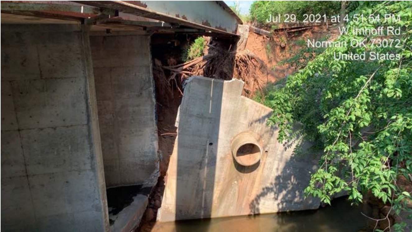
Imhoff Road Bridge over Imhoff Creek – July 29, 2021
