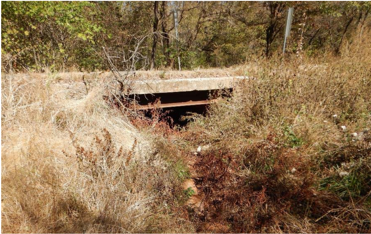
E. Robinson Street Bridge (located east of 72 nd Ave NE).
