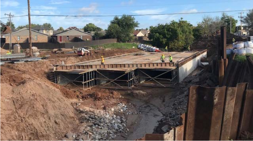
Bridge Replacement – Main Street Bridge over Brookhaven Creek – 2018. $4,905,000.00
