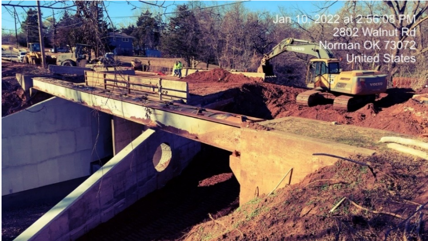
Bridge Rehabilitation– Imhoff Road Bridge emergency repairs – 2020 $1,945,803.59
