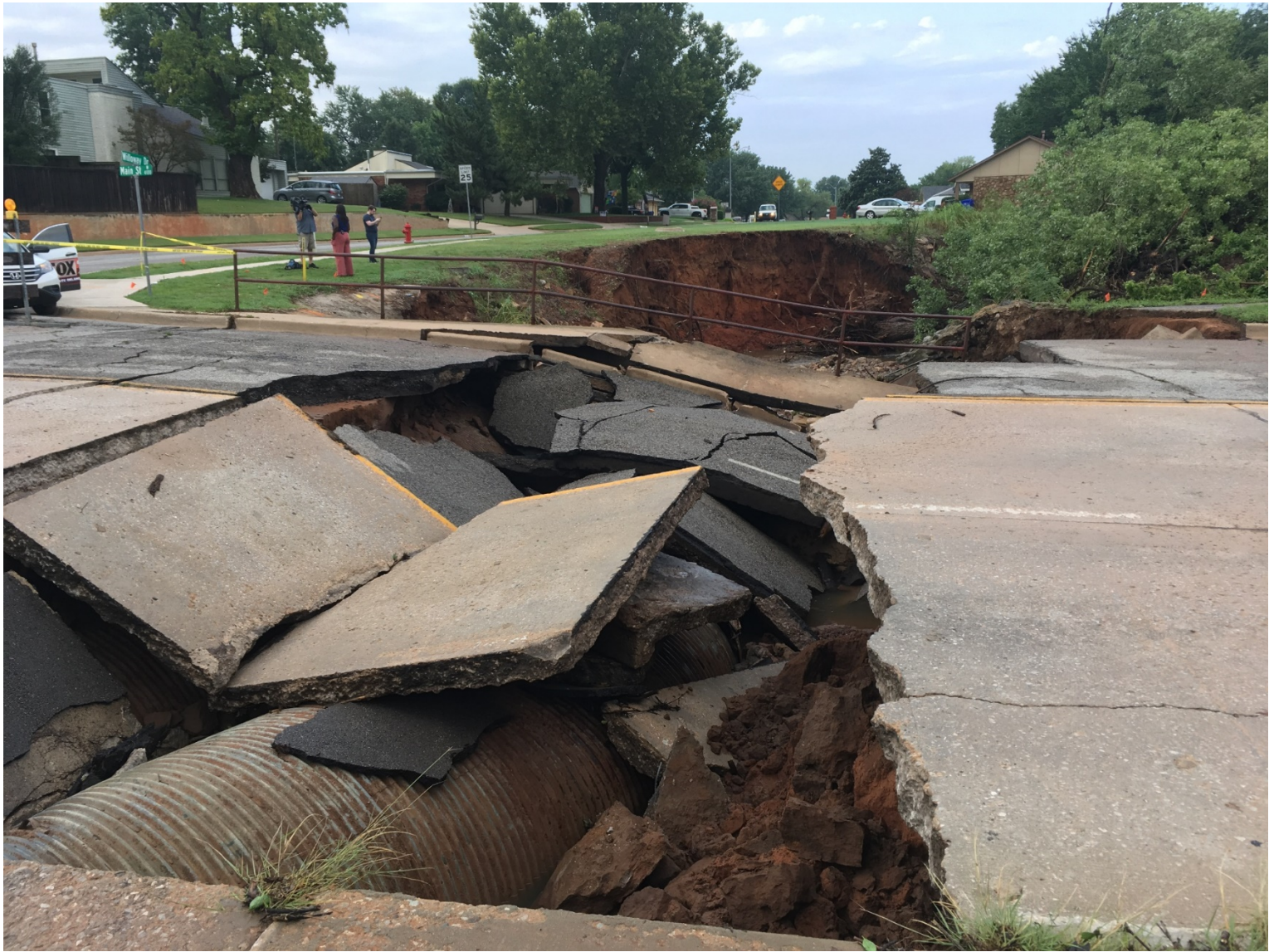
Main Street Bridge over Brookhaven Creek – August 14, 2018.
