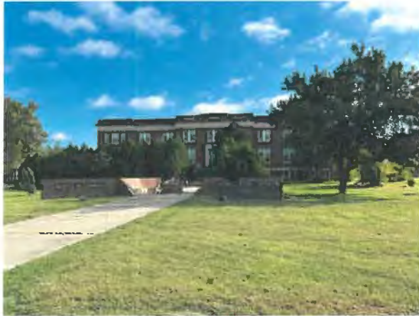
Old Administration Building Preservation
