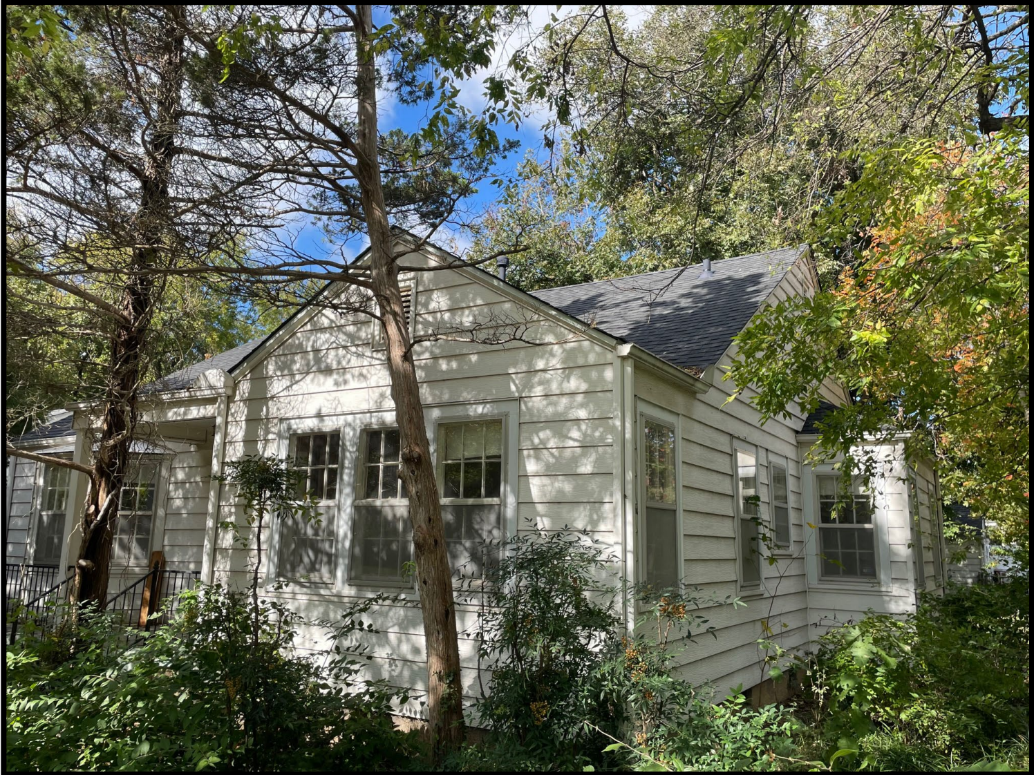
SE Corner of Home Front/Side Yard
