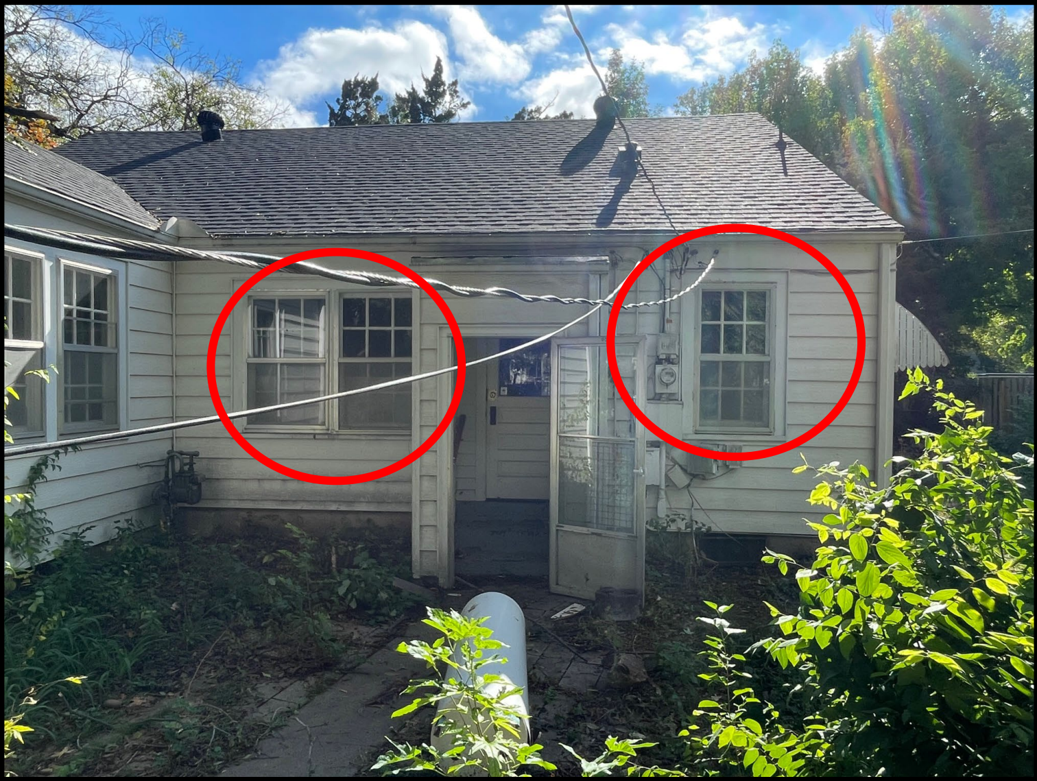
Remove & Reuse 3 Windows on Addition
