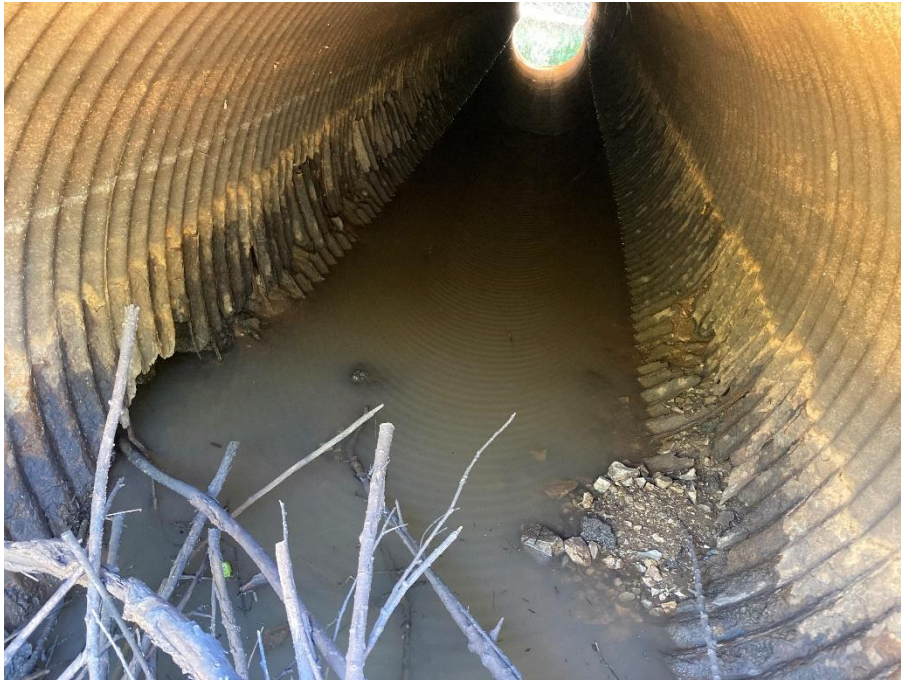
5 perforations in east pipe
