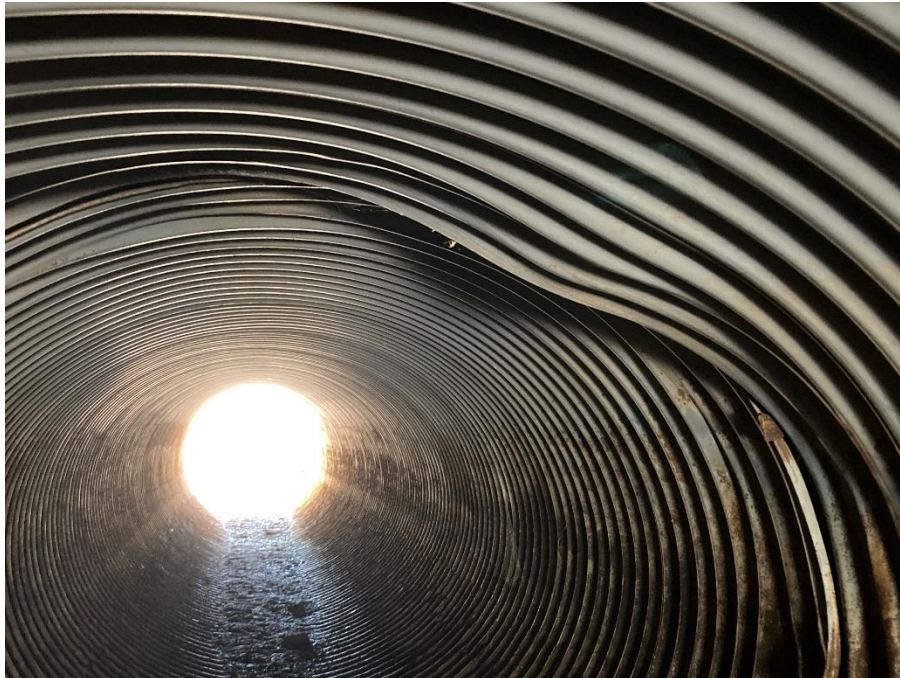
E. pipe 20.5' from north end 3" deflection
