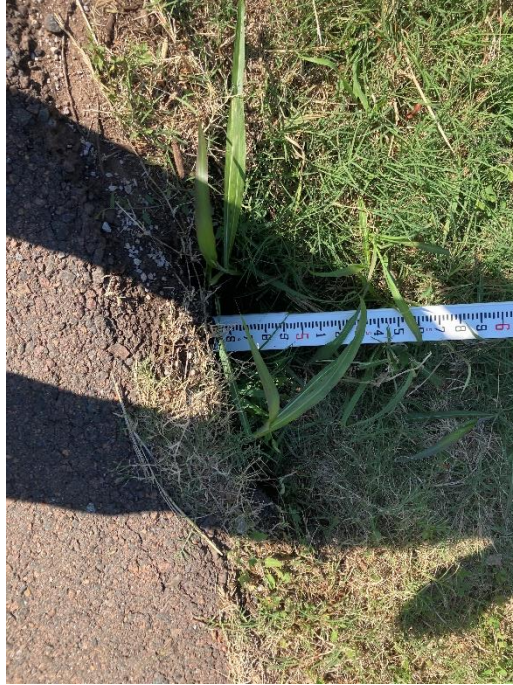
Erosion 4.5' under asphalt with 2' deep void
