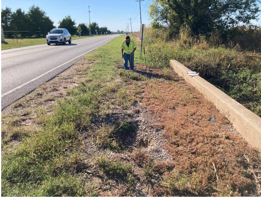
3 sink holes behind north headwall, approx. 1' deep
