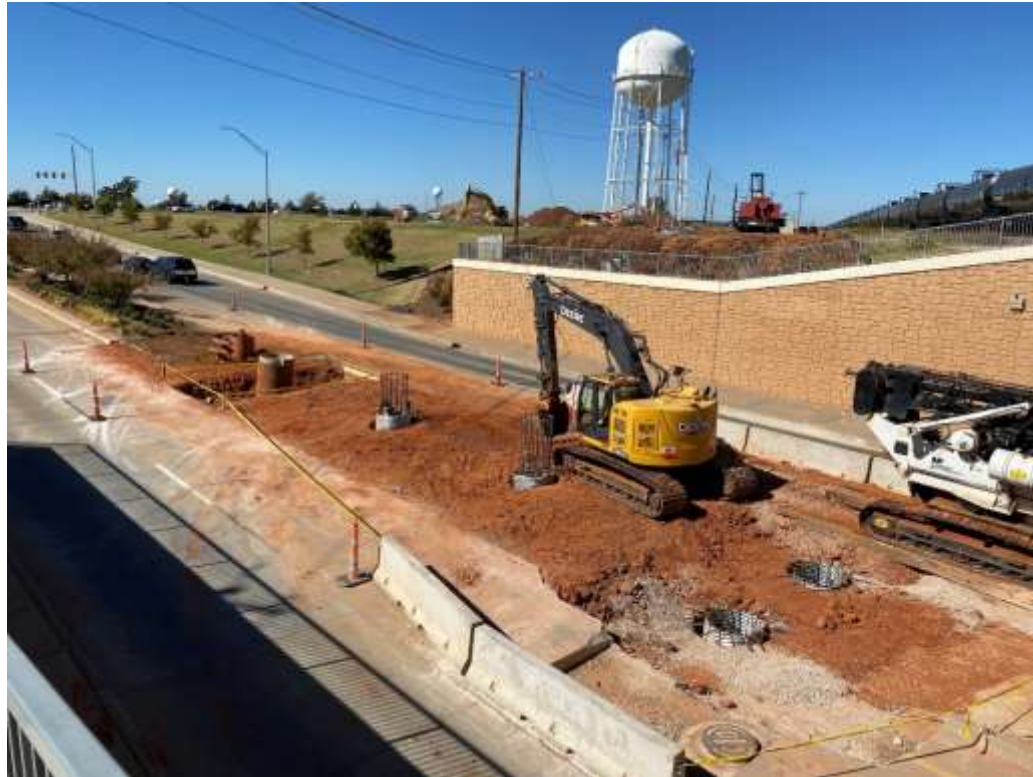
Robinson Street looking northwest at bridge substructure
