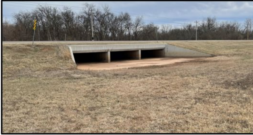
Figure 1. Culvert over Boggy Creek at location BG1.
