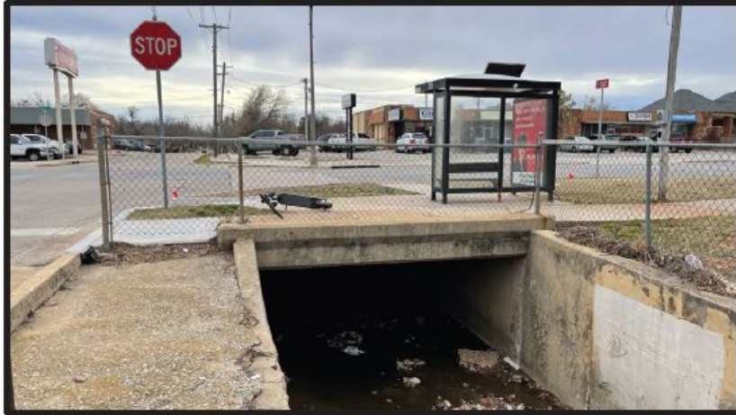
Figure 1. Culvert over Imhoff Creek at location I1.
