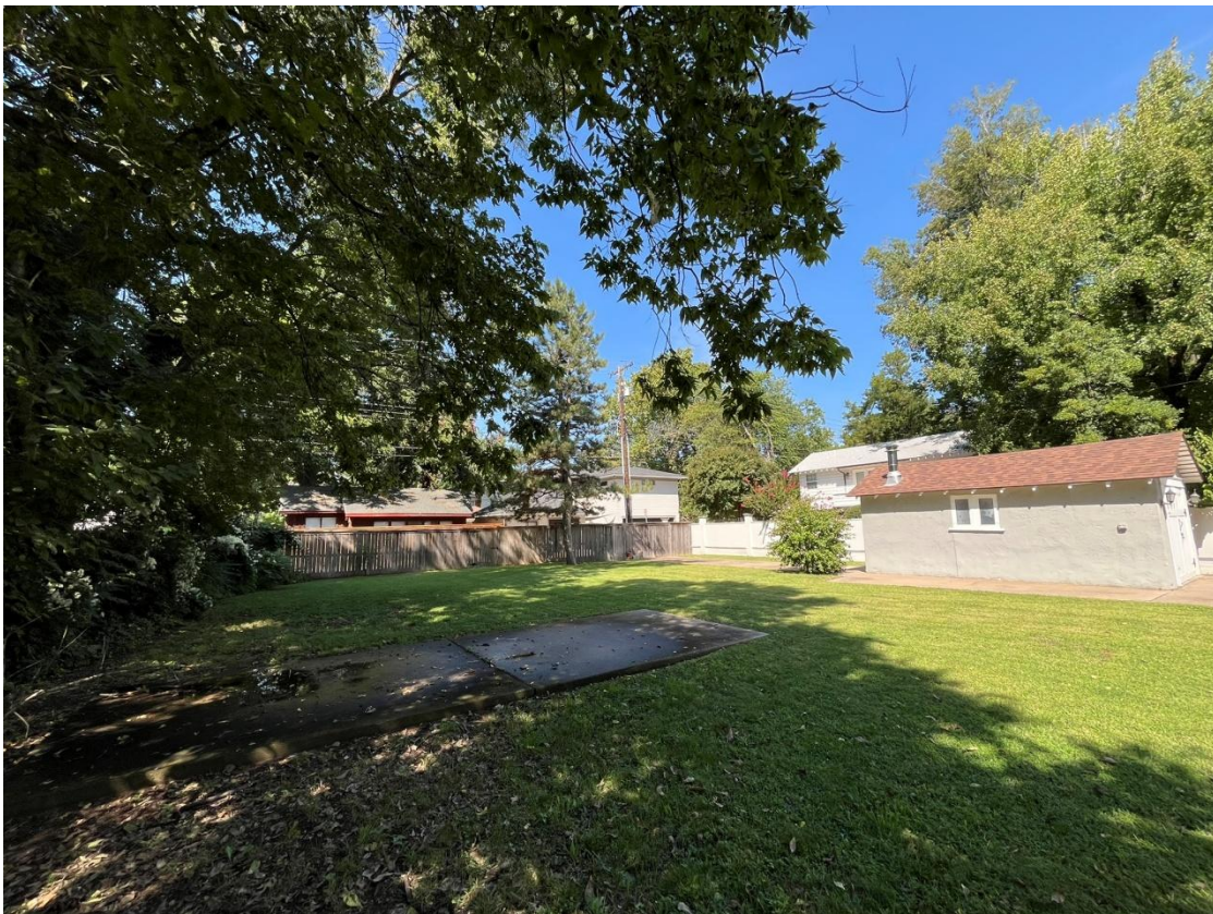
CONCRETE TO BE REMOVED
