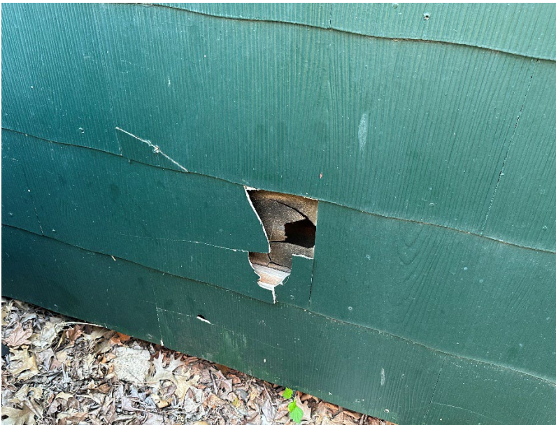
Damaged siding on north side of home
