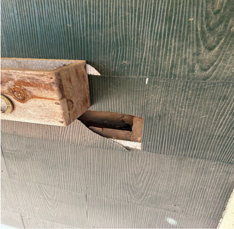
Damaged siding on porch
