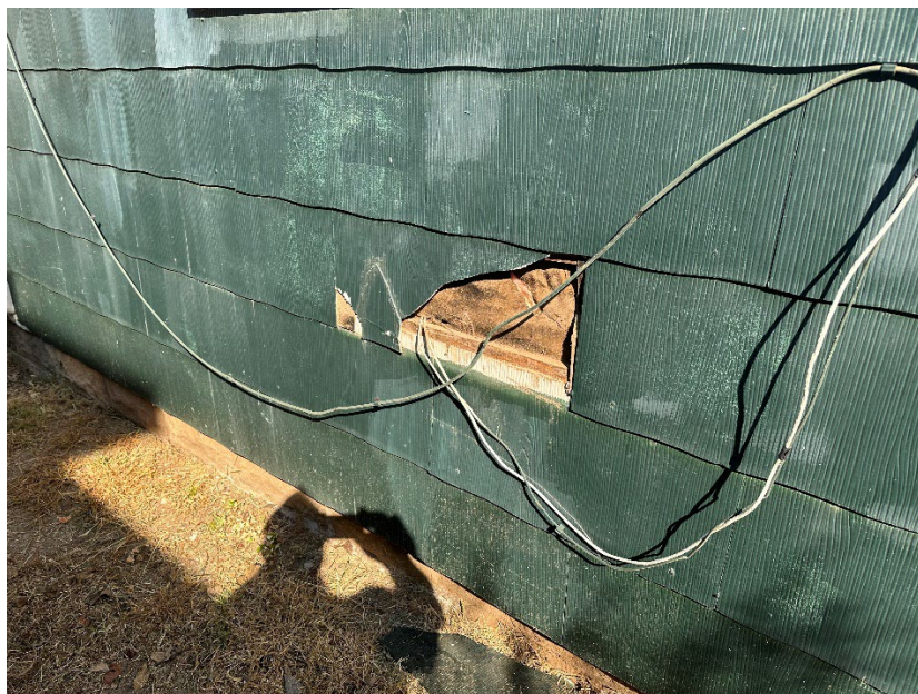
Damaged siding on south side of home
