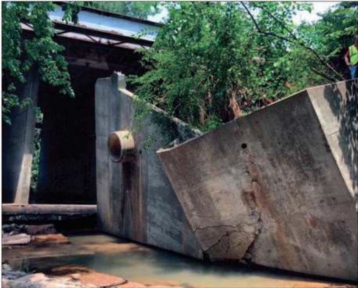
Figure 5: Failure of Wingwall on Imhoff Rd Bridge
