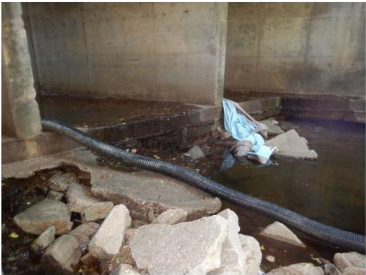
Figure 4-1: Scour at the south end of the structure at Imhoff Road
