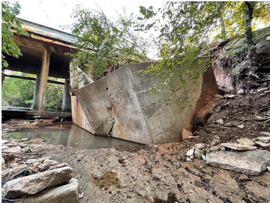
Figure 4-3: Failure of the southeast wingwall of the structure at Imhoff Road
