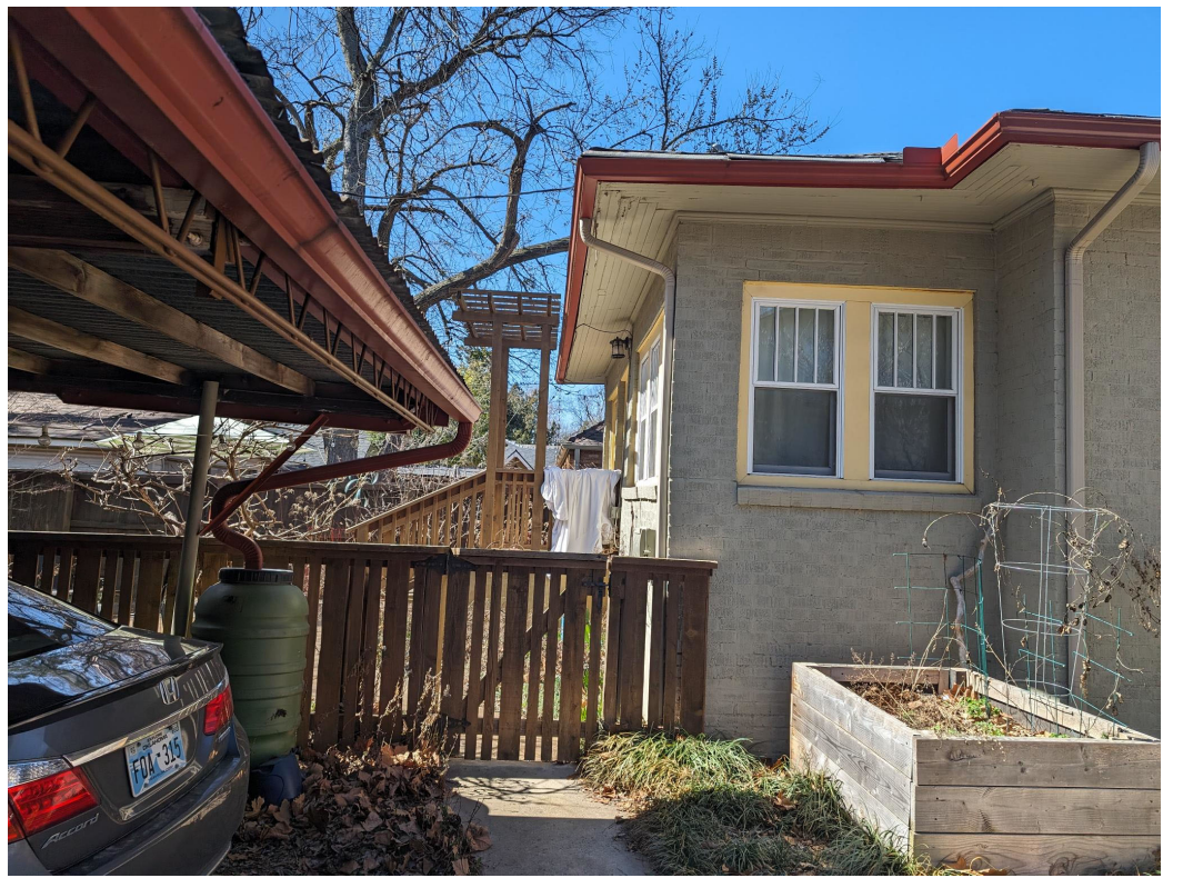
VIEW OF SOUTH SIDE (TOWARDS BACK DOOR)
