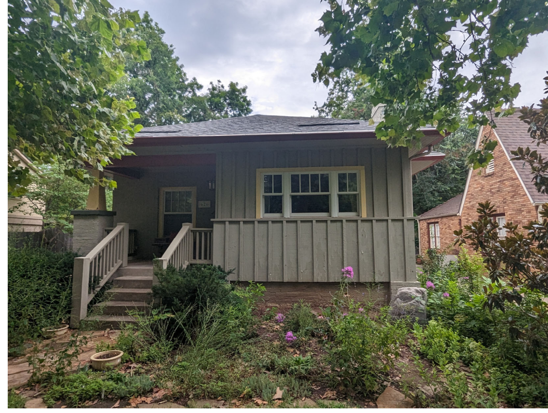
FRONT OF HOUSE (NORTH SIDE)
