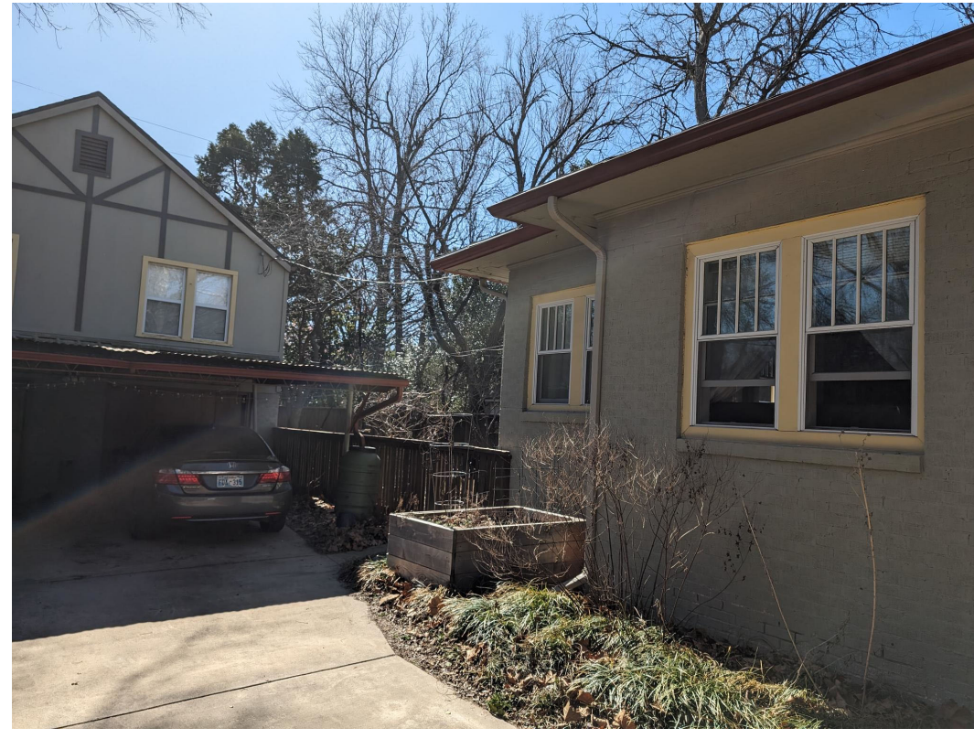
EAST SIDE OF HOUSE/GARAGE (LOOKING SOUTH)
