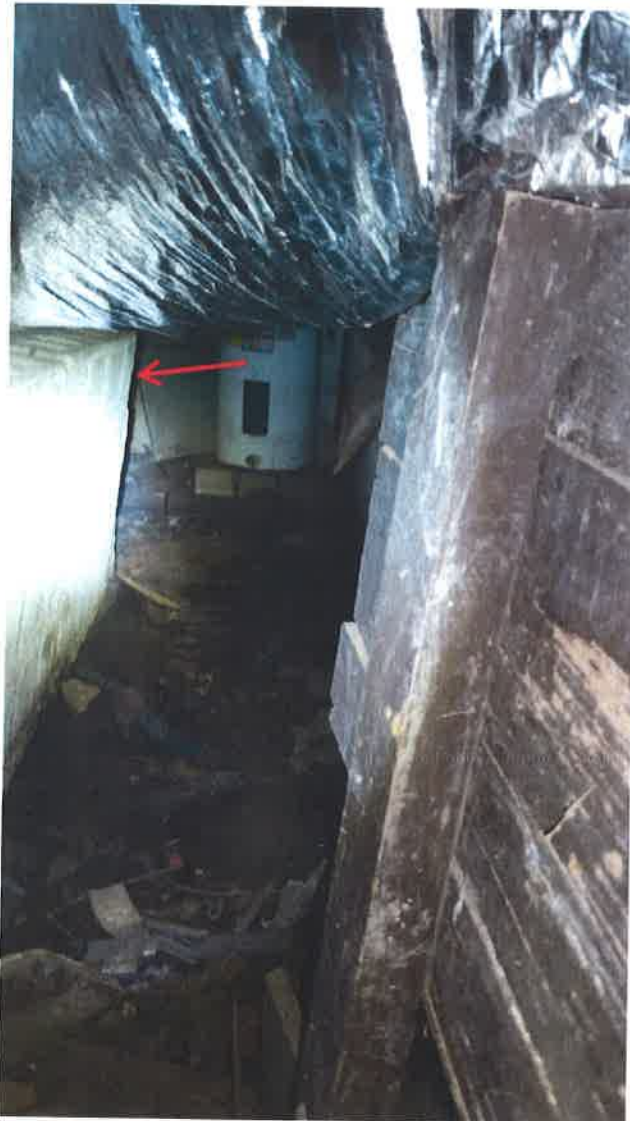
Leaning support wall, moist flooring.
