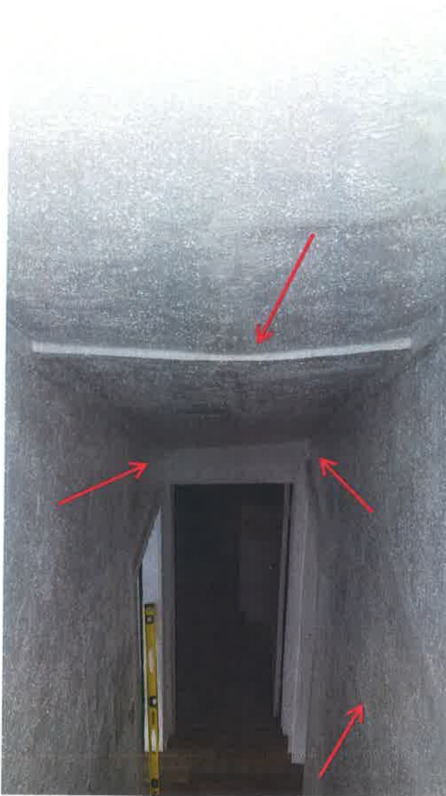
Sagging ceiling in staircase.
