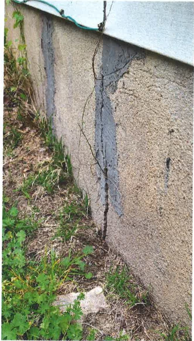
Cracks and displaced stem-wall.
