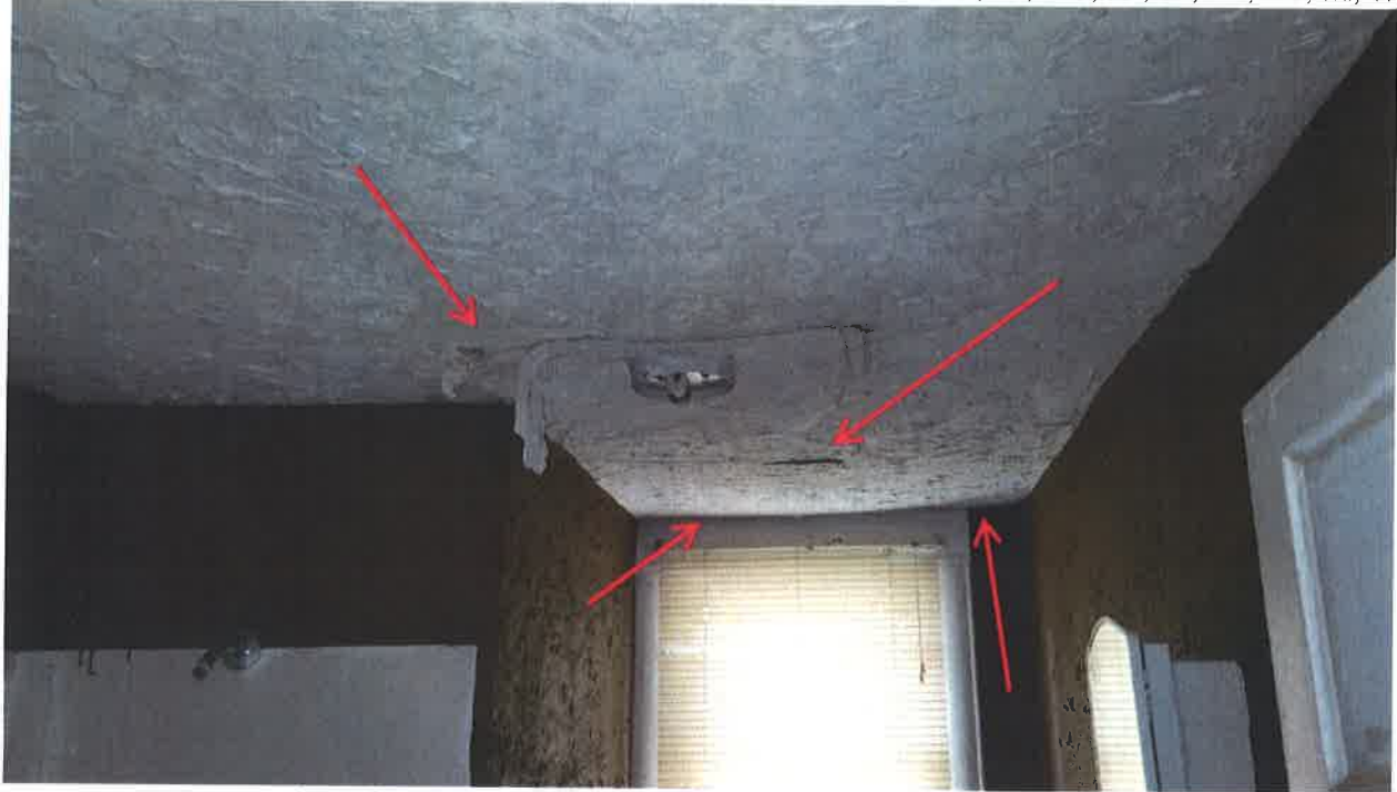
Sagging and crooked ceiling in downstairs bathroom.
