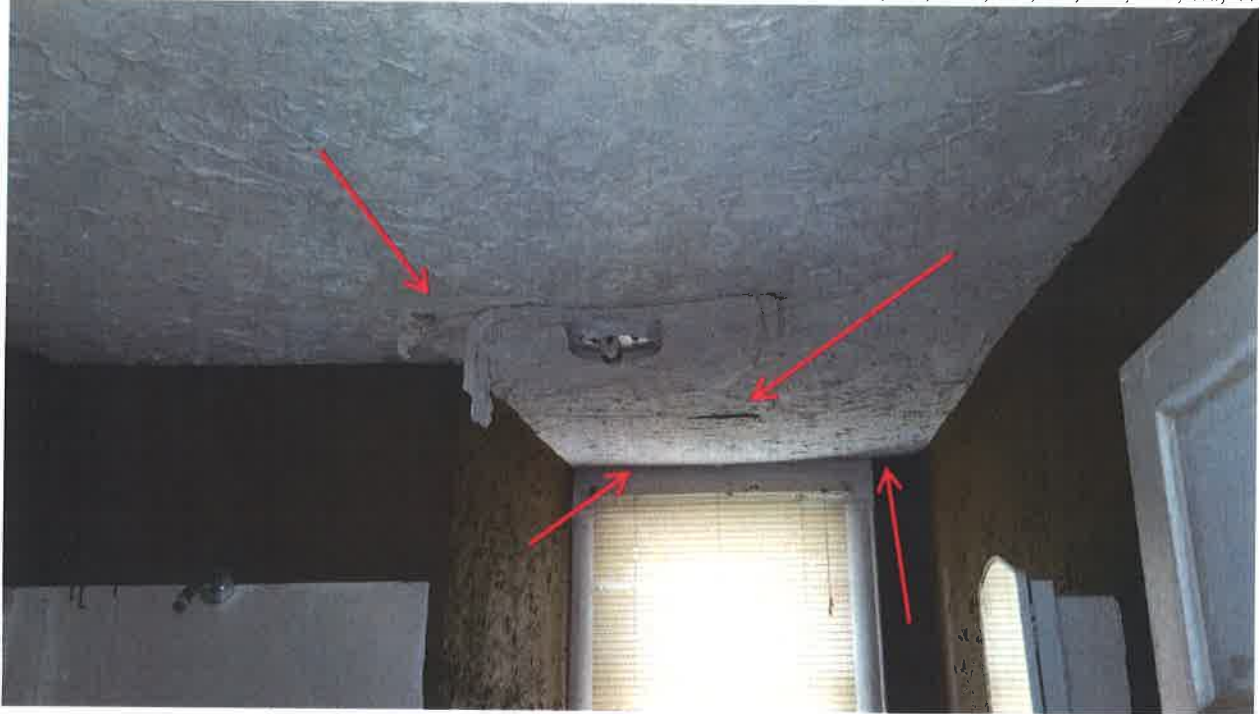
Sagging and crooked ceiling in downstairs bathroom.
