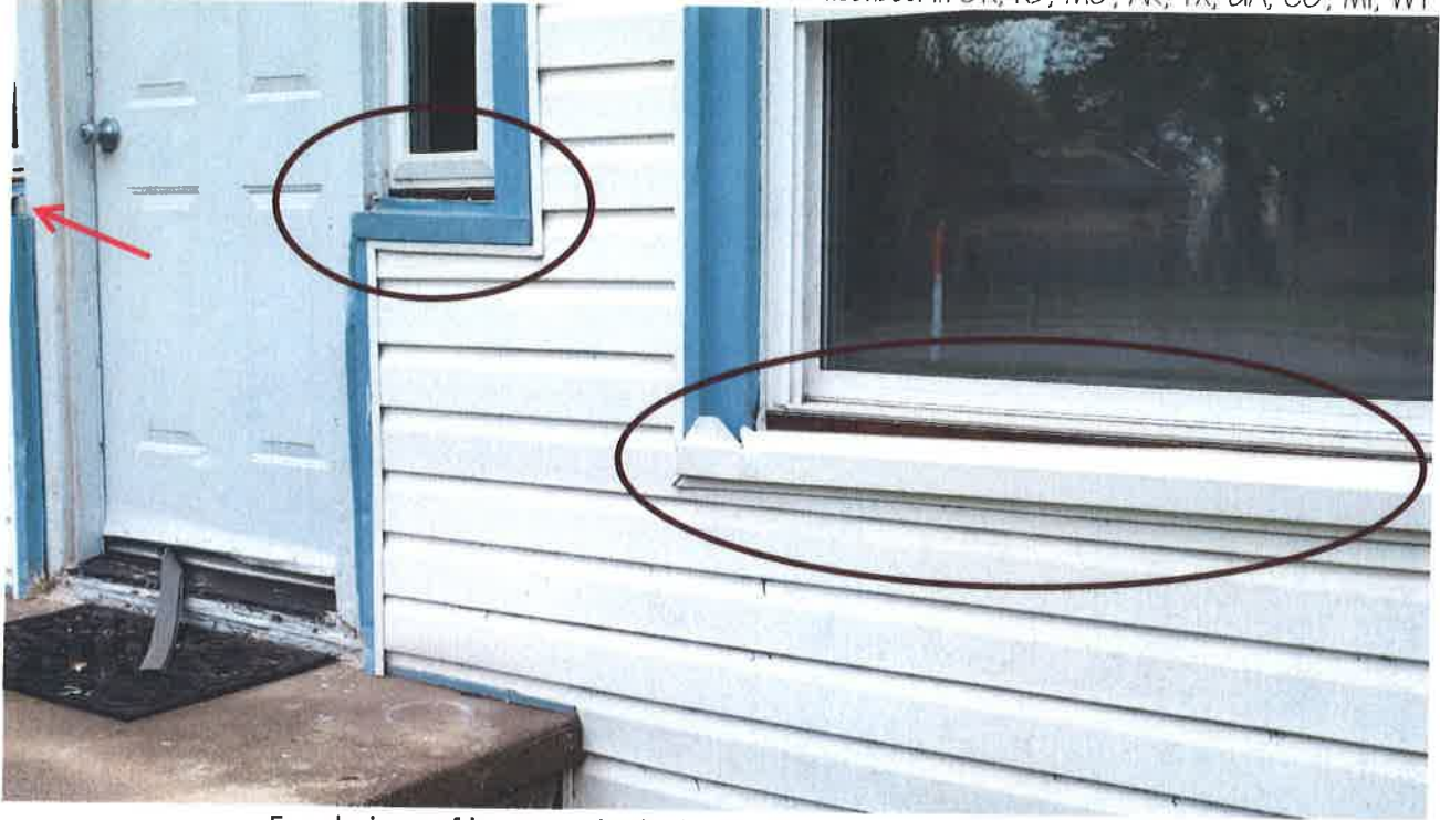
Front view of incorrect windows and poor trim attachment.
