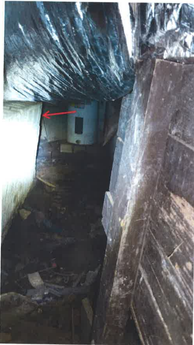
Leaning support wall, moist flooring.
