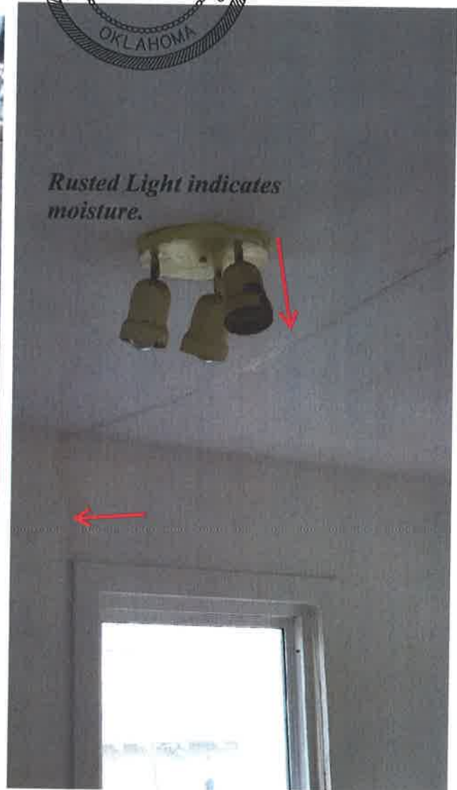
Sagging ceiling and cracks.
