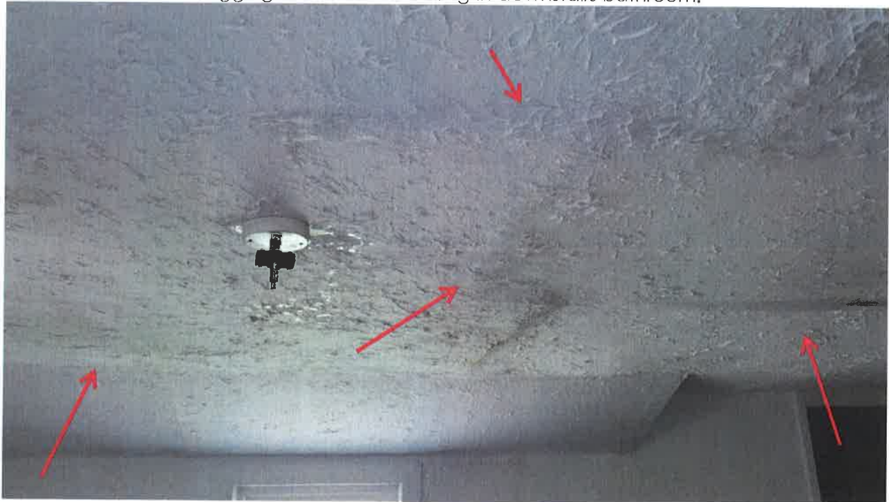
Sagging and crooked ceiling.
