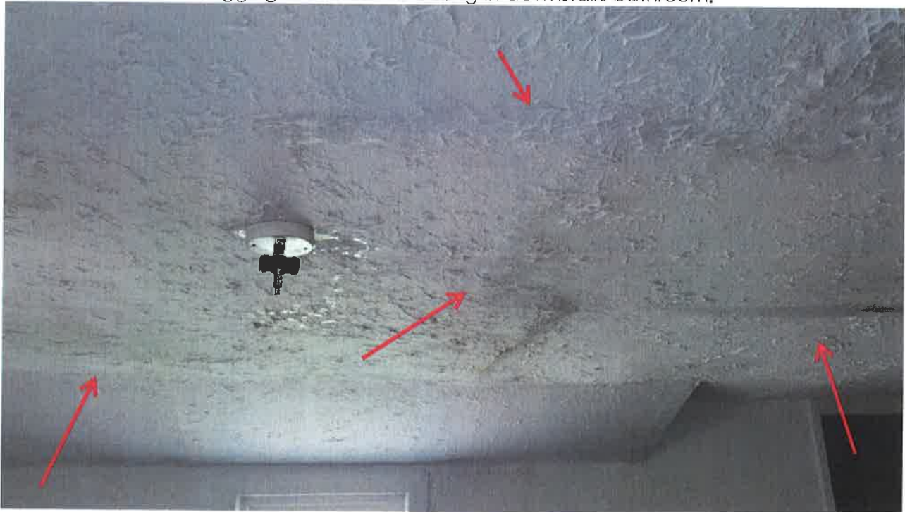
Sagging and crooked ceiling.
