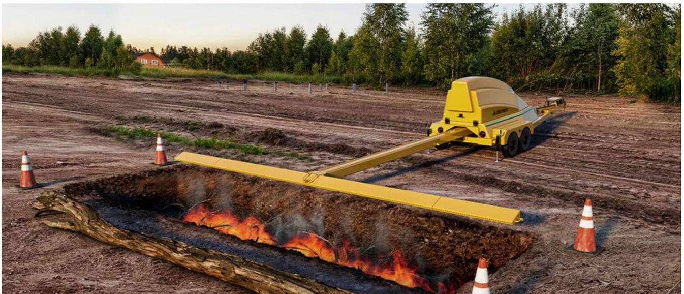
In the areas where surface water and wet conditions are present, the contractor may dig shallower burn pits and utilize berms around the perimeter as shown in the example below....
