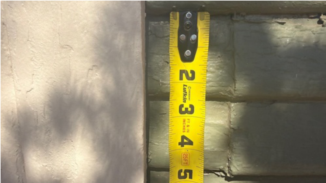
Siding details of existing home
