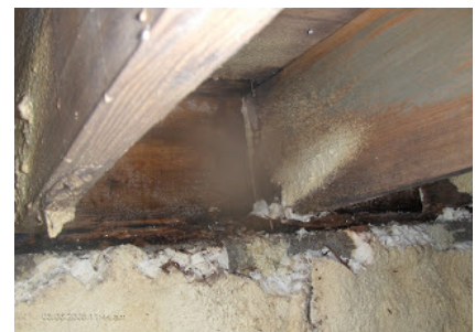
Spray insulation is not recommended since it can trap moisture and mask water leaks, causing wood to rot.
