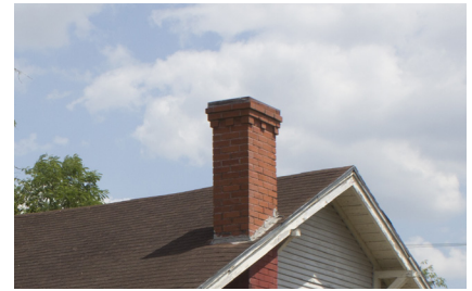
Corbelled chimney cap
