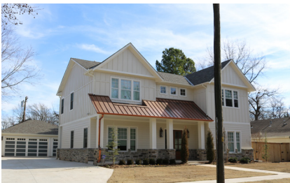
Metal roof on front porch.
