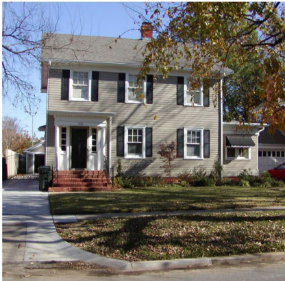
Wood siding, also known as weatherboard, is very typical on historic structures in Norman.
