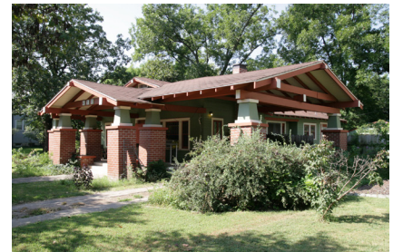
Brick has an inherent natural color and should not be painted or sealed.
