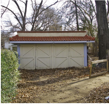
This Mission Revival-style, two-car garage is associated with Patricio Gimeno House in the Chautauqua District.
