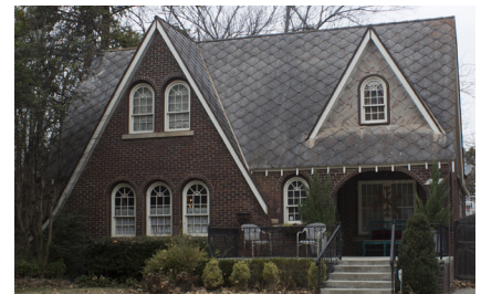
Pressed metal shingle roofing
