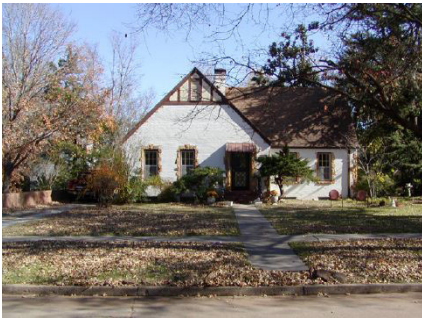
Stucco and half-timbering convey a cottage like atmosphere on this Tudor Revival structure.
