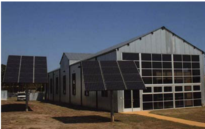
Free-standing solar panels have been installed where they are visible but appropriately located at the rear of the property and compatible with the character of the building. (Source: NPS)
