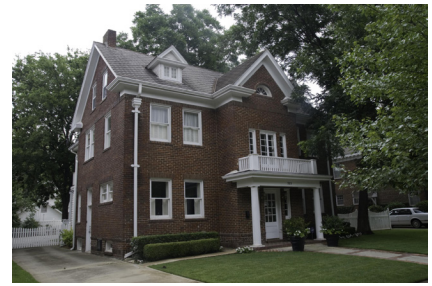
This Colonial Revival-style masonry structure has a wood porch with a roof line balustrade.
