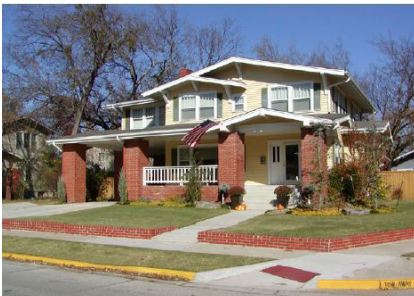
Multiple, low-slung roof planes are very characteristic of Craftsman structures.
