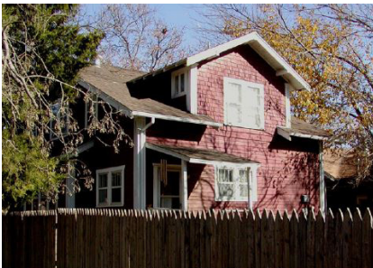
The rear of this Craftsman shows how many roof planes can be used in a single structure.
