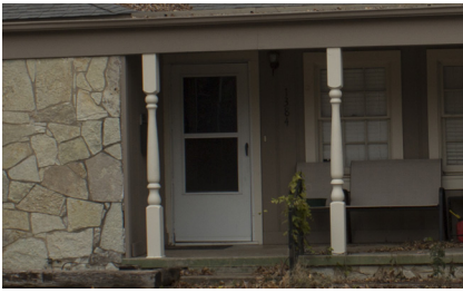
Turned wood posts
