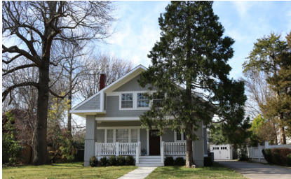
Asbestos shingle siding.
