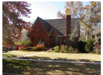
Tudor Revival structures often have steeply pitched roofs and front elevation chimneys.
