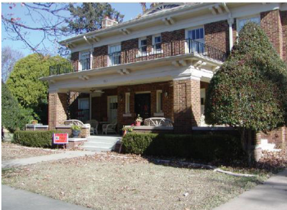
This Italian Renaissance structure has a partially enclosed porch with massive masonry columns.
