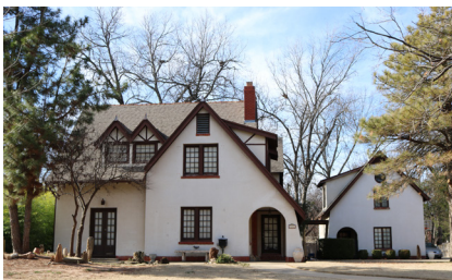
Stucco siding is commonly used on Tudor Revival style houses.
