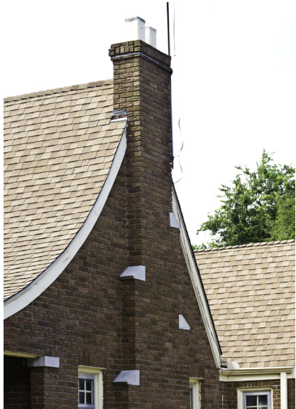
Chimneys are most commonly located on a side elevation of a structure.
