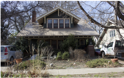
Metal roof replacement on Bungalow.
