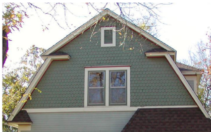
Gable returns highlighted by a multi-color paint scheme are very attractive details on a front gable, gambrel roof structure.
