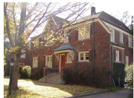
Masonry details such as bond pattern and copings articulate style and design.
