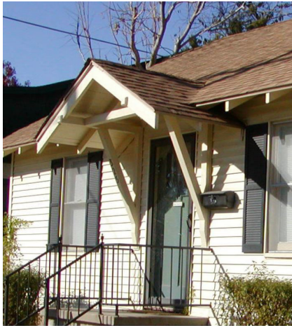
A gable supported by wood braces provides a decorative covered entrance on this National-style structure in the Miller District.
