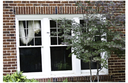
Triple windows are also common especially on front and southern elevations.
