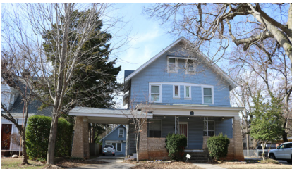
Cut stone piers and columns.
