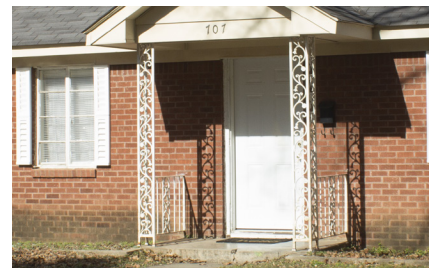
Fabricated metal column
