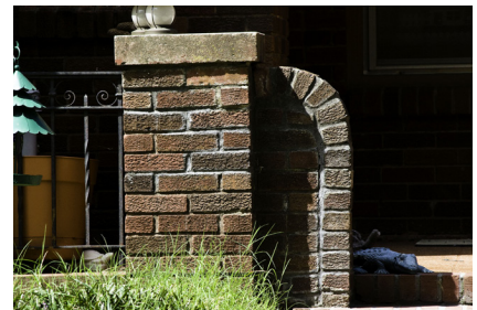
This porch has brick columns with a decoratively curved masonry return wall.
