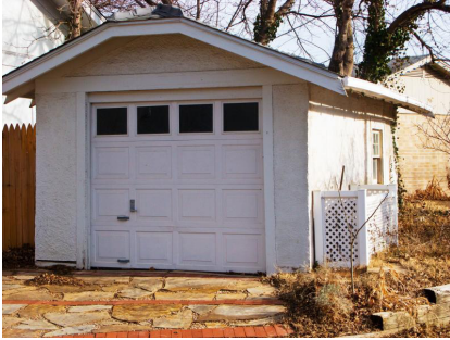
Design details such as the jerkin head gable of this garage are often used as complements to the primary structure.
