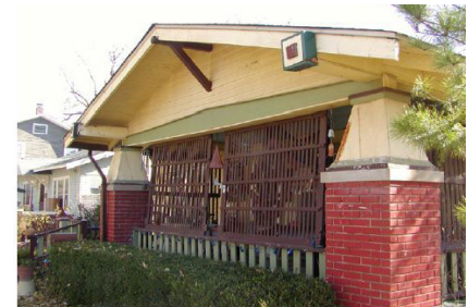
This Craftsman bungalow has a partial front porch with massive brick piers topped by short, elephantine columns.
