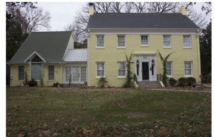
The repainting of previously painted masonry is encouraged over attempts to remove the paint films chemically or abrasively.
