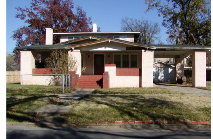
Stucco walls and porch piers give this Mission Revival style Bungalow its distinctive character and should be preserved.
