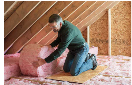
Fiberglass batt is an appropriate insulation material.
