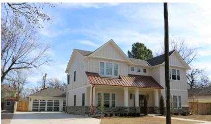
Contemporary house with stone skirting.
