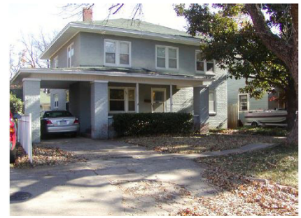
On this Prairie style structure, a partial front porch extends into a porte cochere, meaning literally “a carriage door.”
