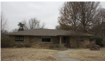
Cut stone siding on Ranch Style house.
