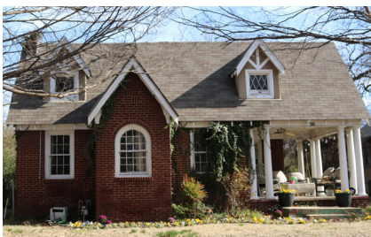
Composition shingle roofing
