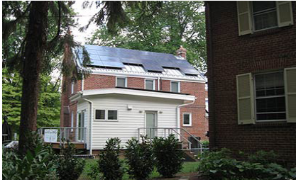
Not recommended - solar roof panels have been installed at the rear, but because the house is situated on a corner, they are highly visible and negatively impact the character of the historic property. (Source: NPS)
