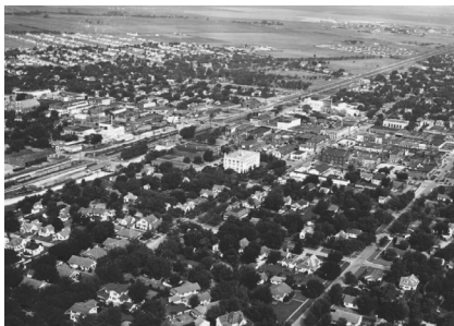
Aerial View of Norman in the 1950s
