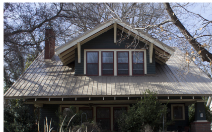
R-panel metal roofing
