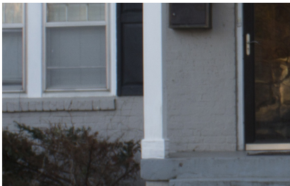
Base of a column
