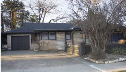
Cut stone siding.
