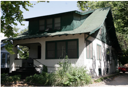
Craftsman-style structures often use multiple materials for exterior walls. This house has a combination of stucco and wood shingles.
