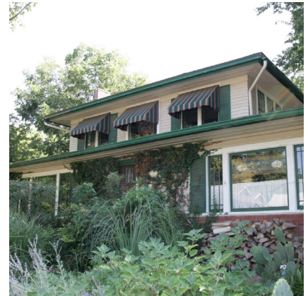
Window awnings may serve as an energy saver by regulating the amount of sunlight entering the structure.
