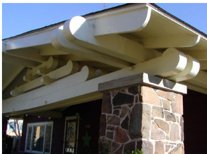
Decorative collar beams spanning a porch gable are characteristic of high Craftsman style.
