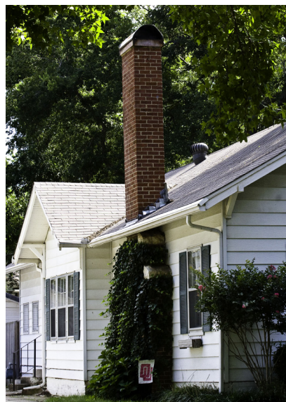
A typical bungalow chimney with a chimney cap.
