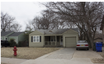
Asbestos shingle siding.
