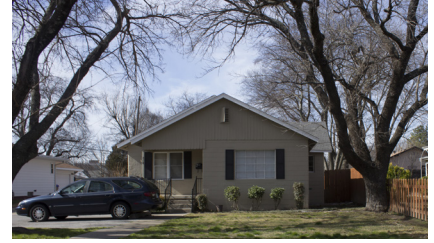
Painted concrete block should remain painted.
