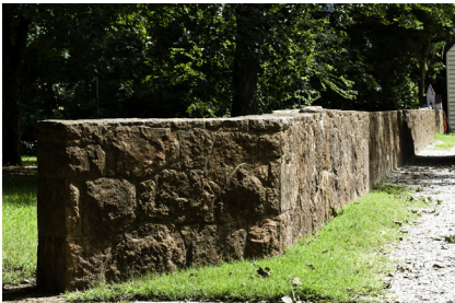
There are few stone walls in Norman’s historic districts so those that exist have special significance.
