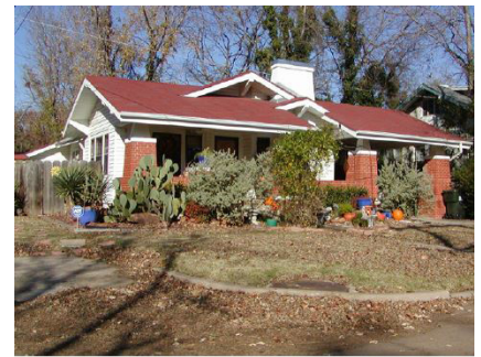
This Mission Revival structure in the Miller District includes a front elevation chimney, a detail borrowed from Tudor Revival style.
