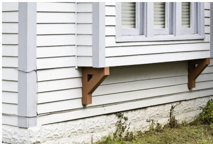
Brackets are sometimes used to support bay windows on bungalow structures.
