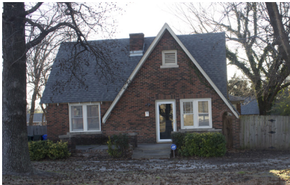
Front facing gable
