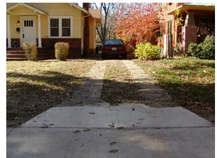
Ribbons or runners are very traditional and generate less runoff than impervious surfaces.
