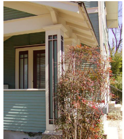
The corner of this Prairie-style porch has a wealth of wood details: molded columns, exposed rafter tails, and massive cross beams.
