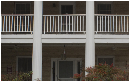
Balustrade along edge of porch
