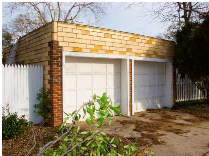
This two-car garage was built around 1944, apparently using leftover building materials.
