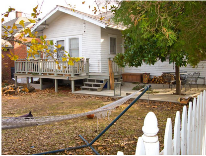
Because of their visibility, decks on corner properties should be designed sensitively to least detract from the original structure.
