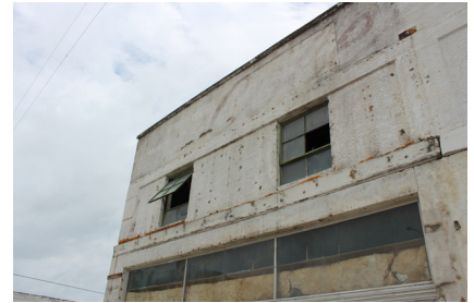
Broken glass should be replaced, and features such as canopies should be replaced where they existed originally.
