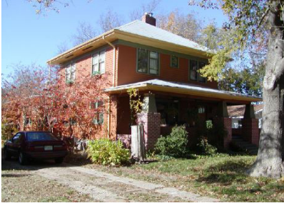
A symmetrical, hipped roof is common on Prairie style structures.
