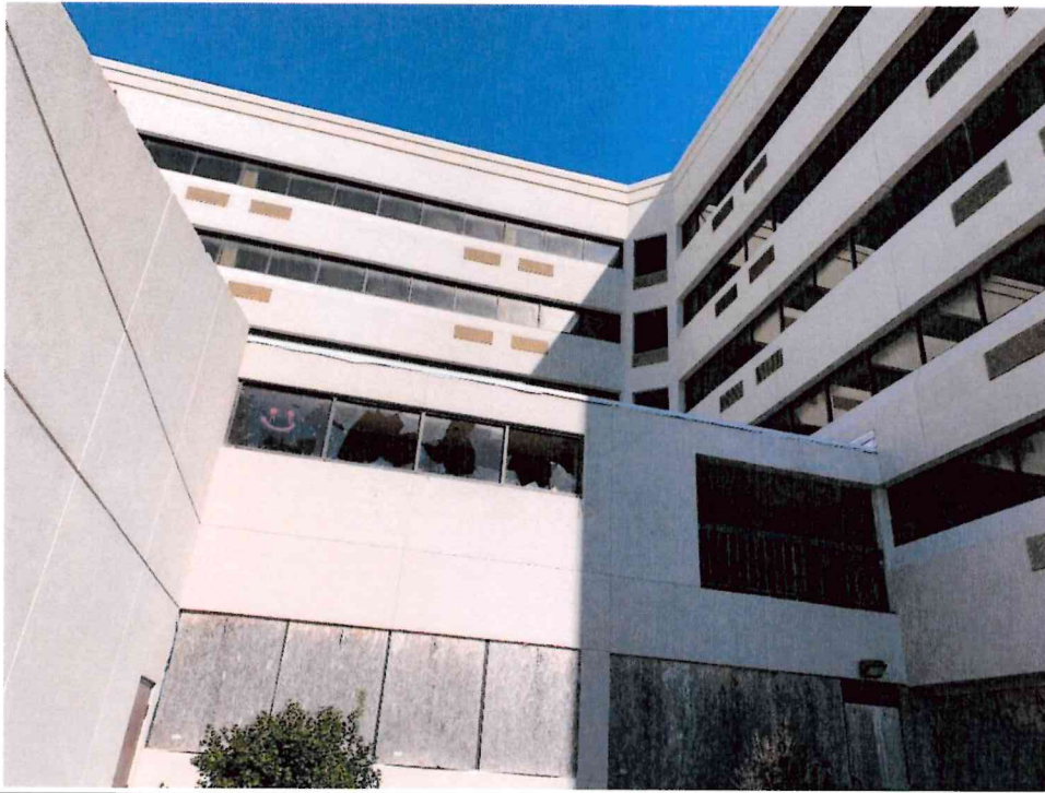
2 nd floor broken windows and 1 st floor boarded windows/doors 1-8-2025
