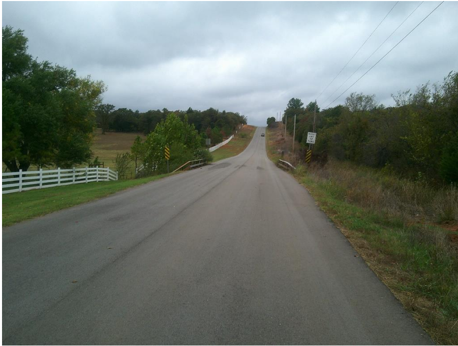
Roadway view, looking west
