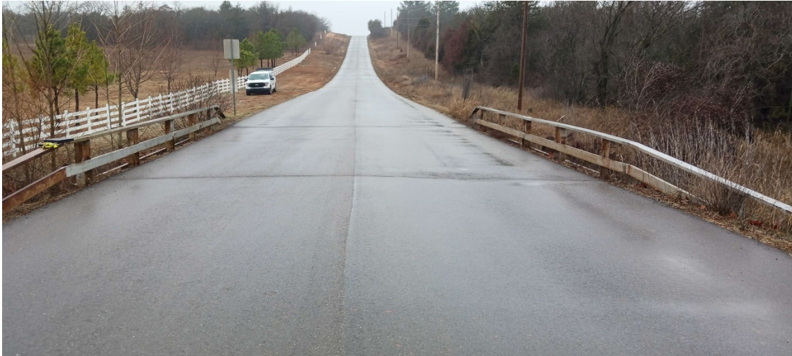
Photo 1. Looking West from Existing Bridge
