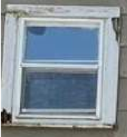
#10. Wood window. Not working. Wood rot.
