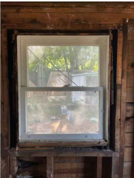
#14. Wood window. Not working, wood rot.
