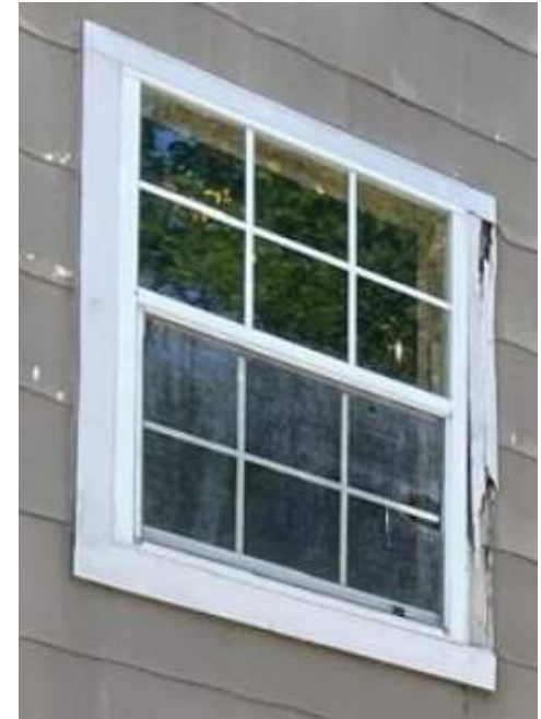
#11. Vinyl window partially working. Wood rot.
