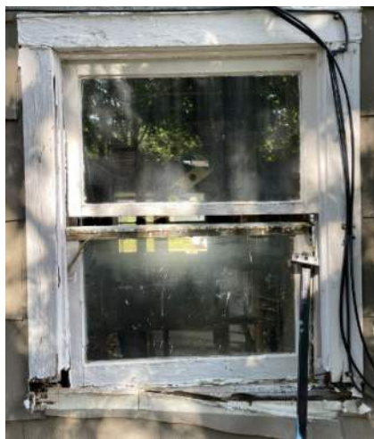
#15. Wood window. Not working, wood rot.
