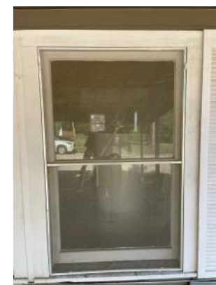
#5. Metal & wood. Does not work. Wood rot.
