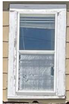
#7. Storm windows over wood-rotten, partially working.
