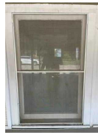
#4. Metal & wood. Does not work. Wood rot.
