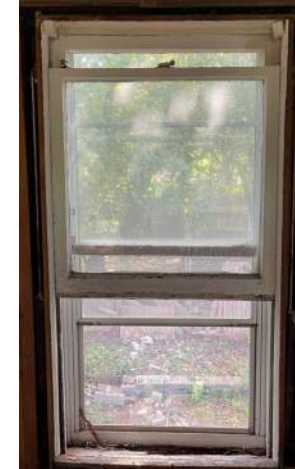
#18. Wood window. Partially working. Wood rot.
