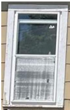
#9. Storm windows over wood-rotten, not working.
