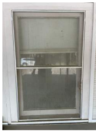
#3. Metal & wood. Does not work. Wood rot.
