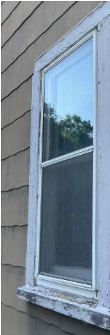
#19. Metal storm windows over wood structure -rotten. Working.
