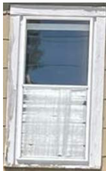
#8. Storm windows over wood-rotten, not working.
