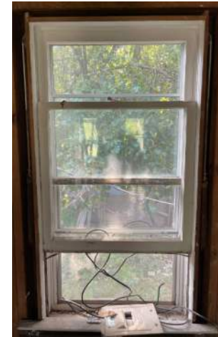
#17. Wood window. Not working, wood rot.
