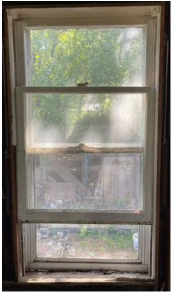
#14. Wood window. Not working, wood rot.
