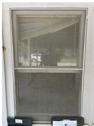
#2. Metal & wood. Partially works. Wood rot.
