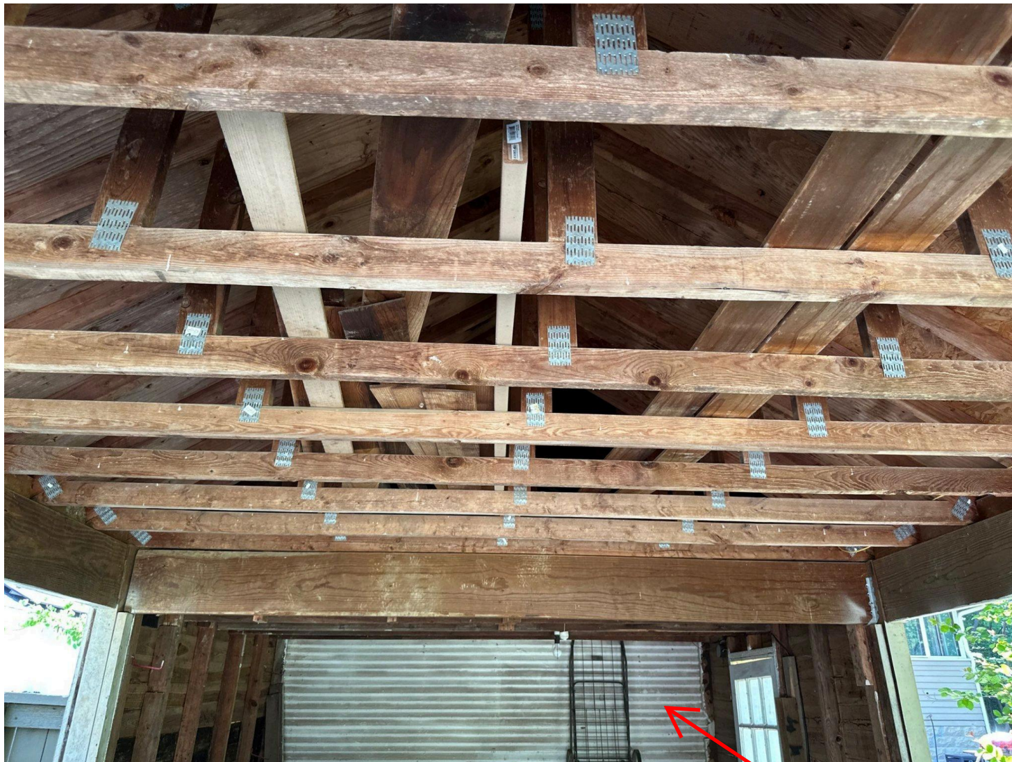
CARPORT "INTERIOR" ROOF STRUCTURE
