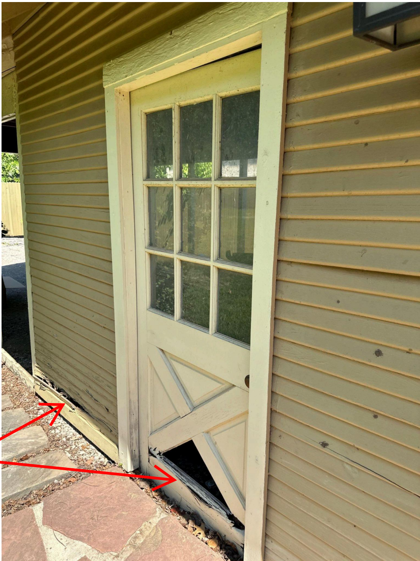
CLOSE UP: DETERIORATED CARPORT PEDESTRIAN DOOR
