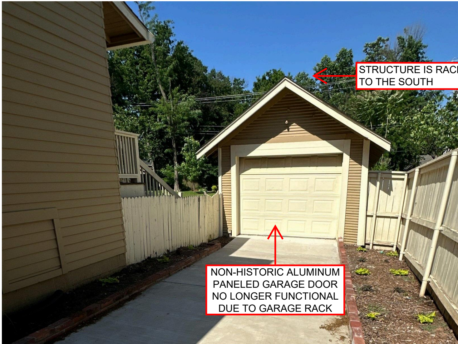
EAST (FRONT) ELEVATION OF GARAGE IN PROXIMITY TO FENCES AND HOUSE
