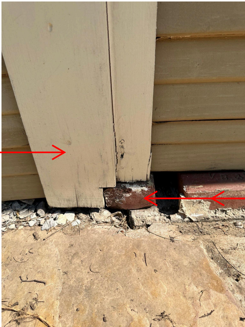
CLOSE UP: SEAM BETWEEN ORIGINAL STRUCTURE (GARAGE; RIGHT) AND HISTORIC ADDITION (CARPORT; LEFT)
