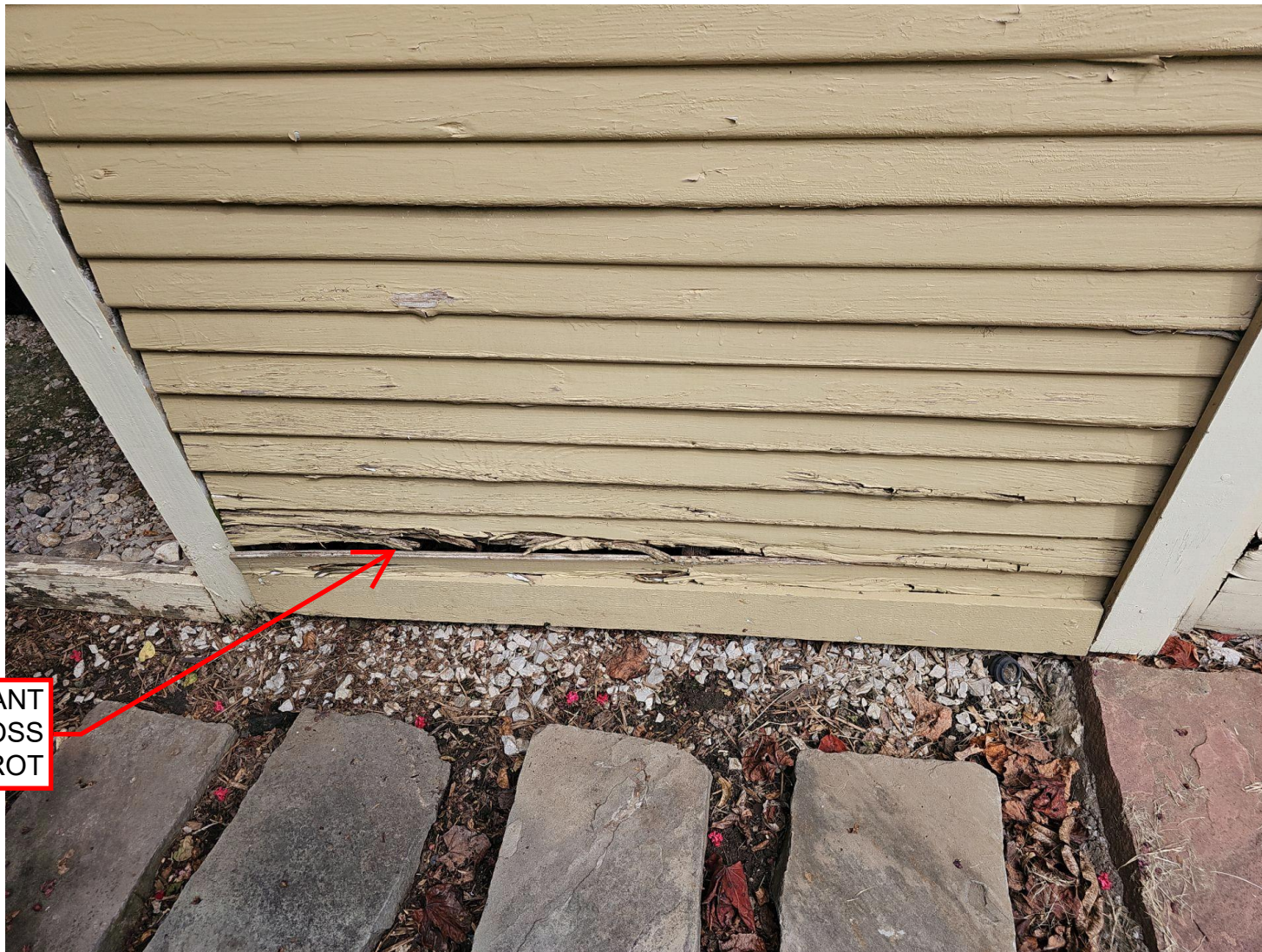
CLOSE UP: DETERIORATED WOOD T-117 (DOUBLE TEARDROP) SIDING
