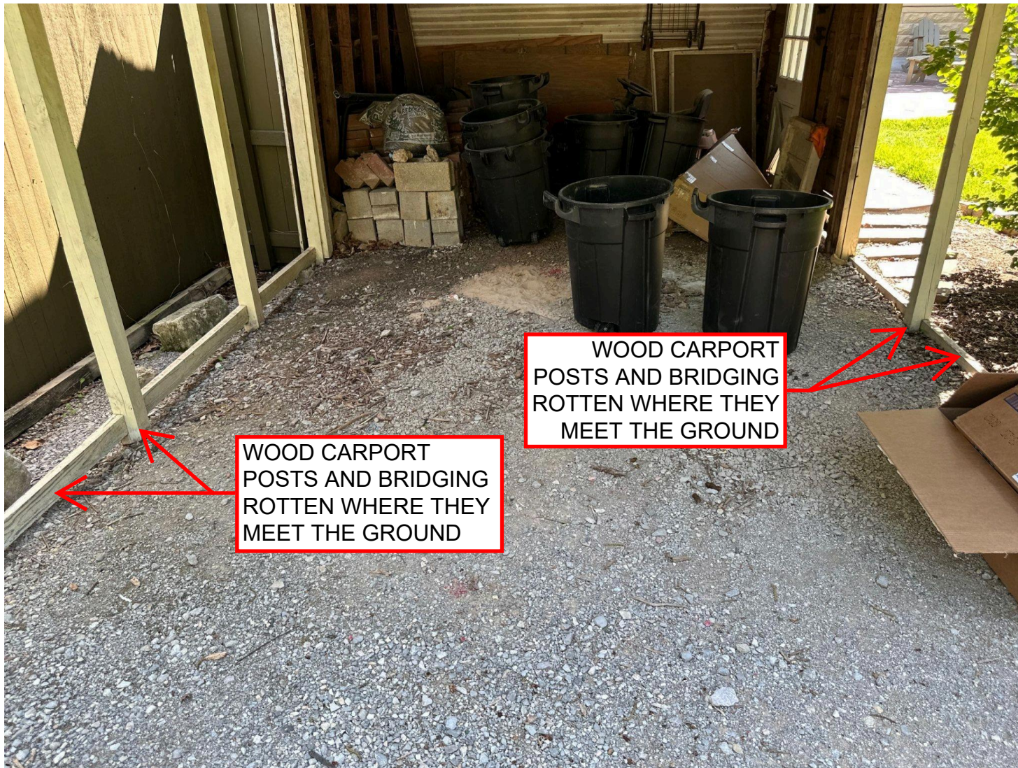
CARPORT "INTERIOR" GRAVEL FLOOR
