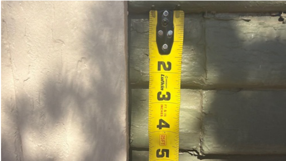
Siding details of existing home
