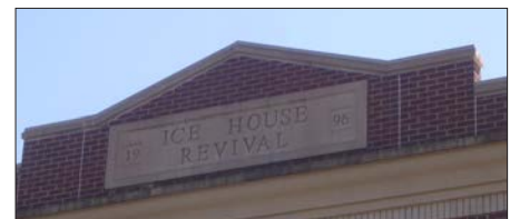
Masonry parapet sign
