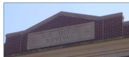
Masonry parapet sign
