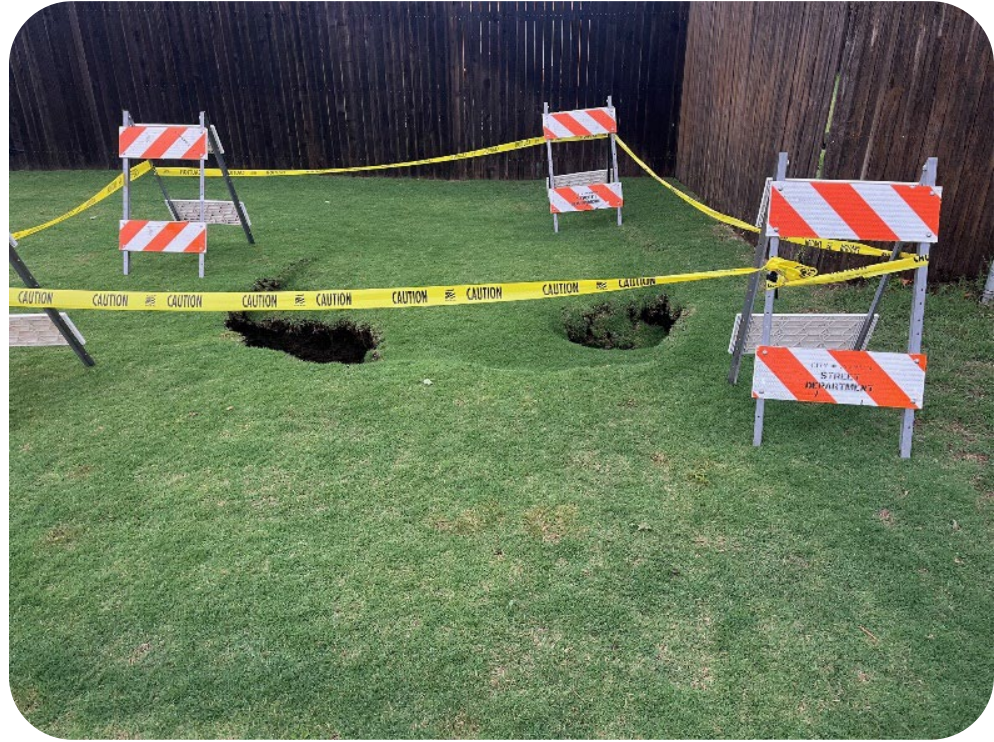
Pipe Failure Causing Sinkholes at Rambling Oaks Drive
