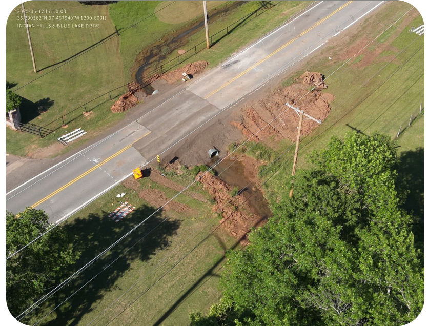
Pipe Washout and Repair at Indian Hills Road and Blue Lake Drive
