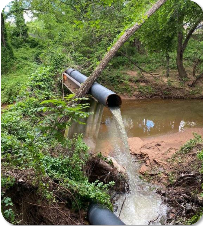
Sewer Failure near 730 Stinson Avenue
