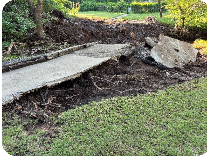
Brookhaven Creek Pedestrian Bridge Collapse
