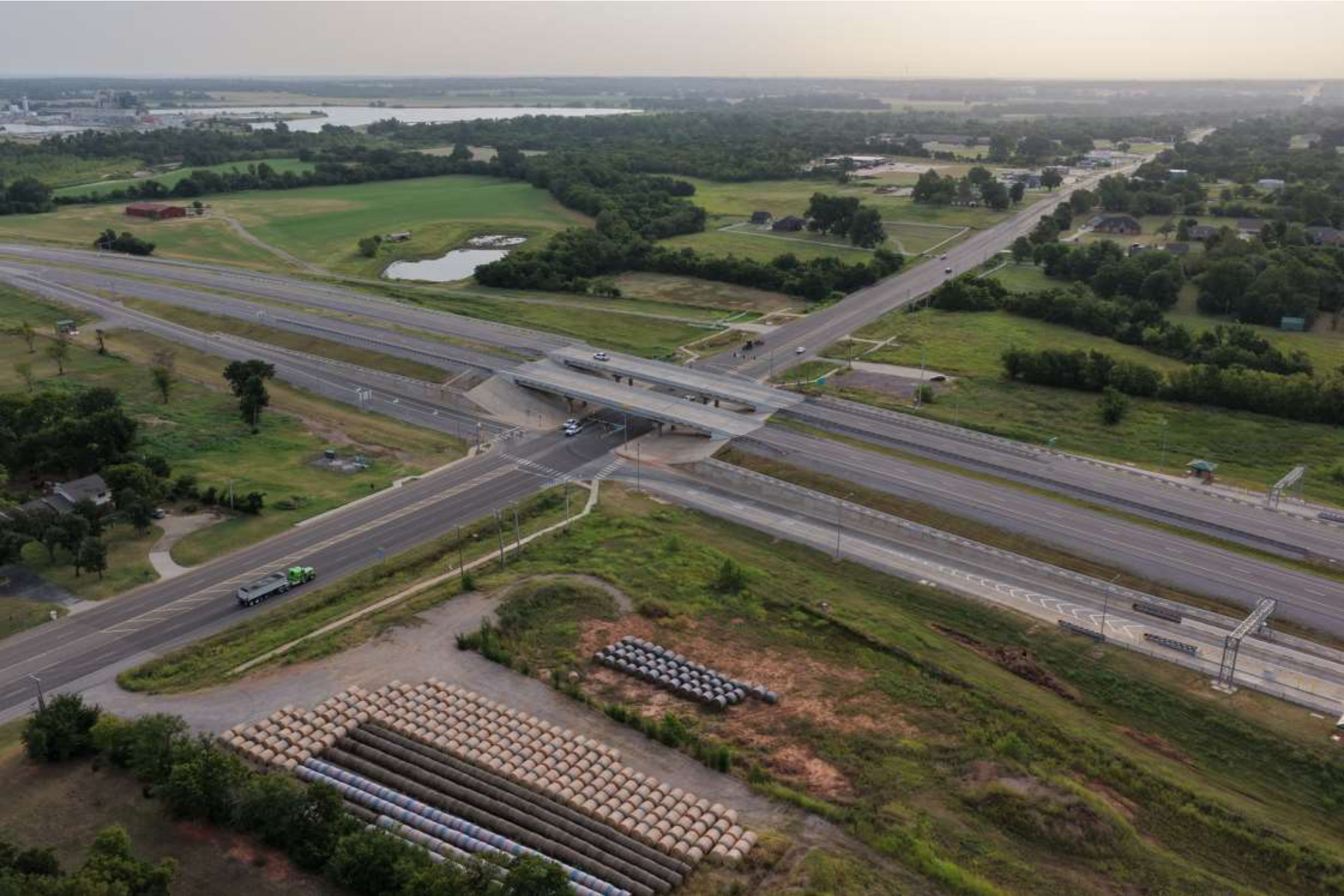
I-335/Kickapoo Turnpike NE 23rd Interchange
