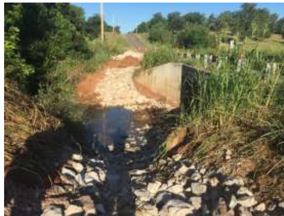
Bridge Maintenance on Cedar Lane
