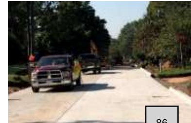
Walnut Road (Urban Reconstruction)
