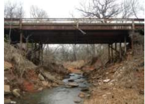
Bridge on 60 th Avenue
