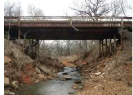
Bridge on 60 th Avenue
