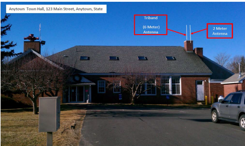
Figure 2. Example of ground-level photograph showing proposed attachment of new equipment.
