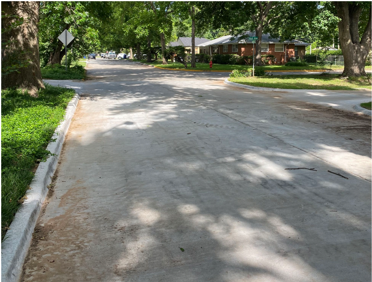
Grover Lane after reconstruction.
