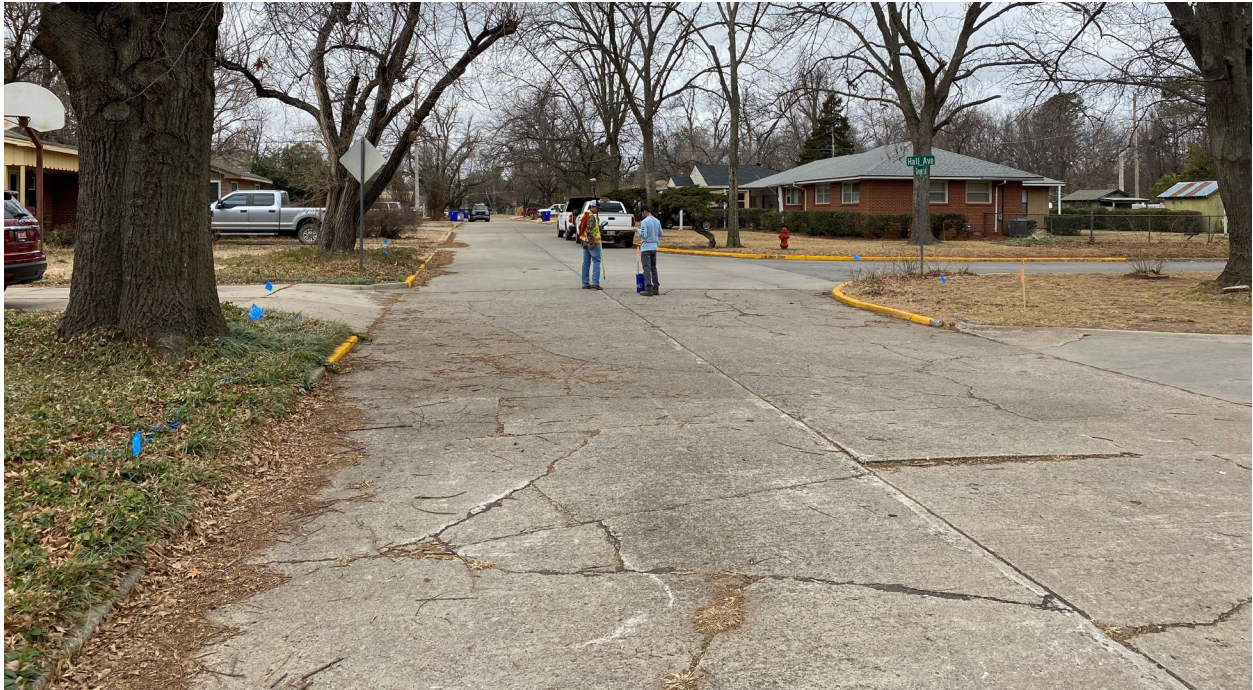
Grover Lane before reconstruction.
