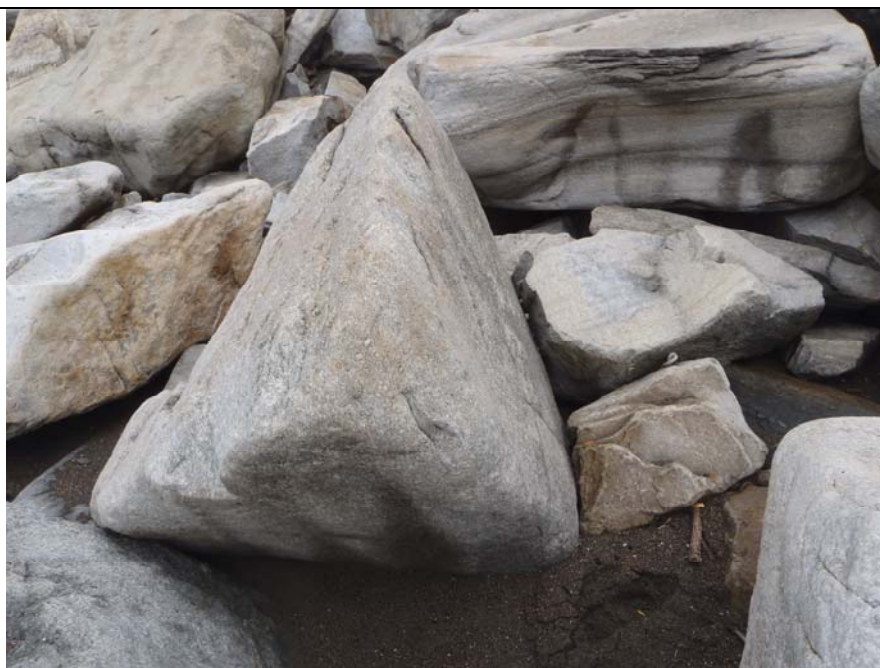
Missing armor—exposed core rock, rounded edges
