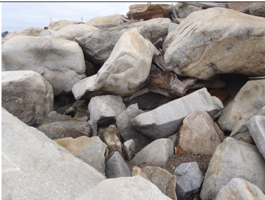
Rounded stones, Missing armor stones
