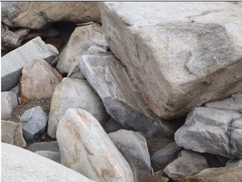
Missing armor units near toe
