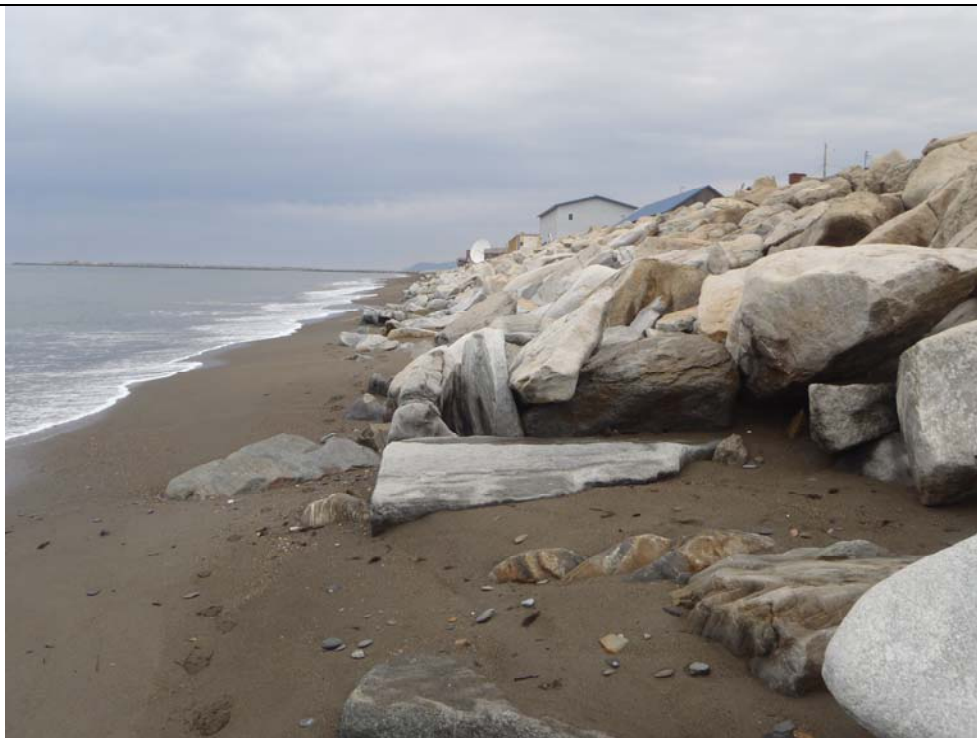
Missing section of toe, rounded edges
