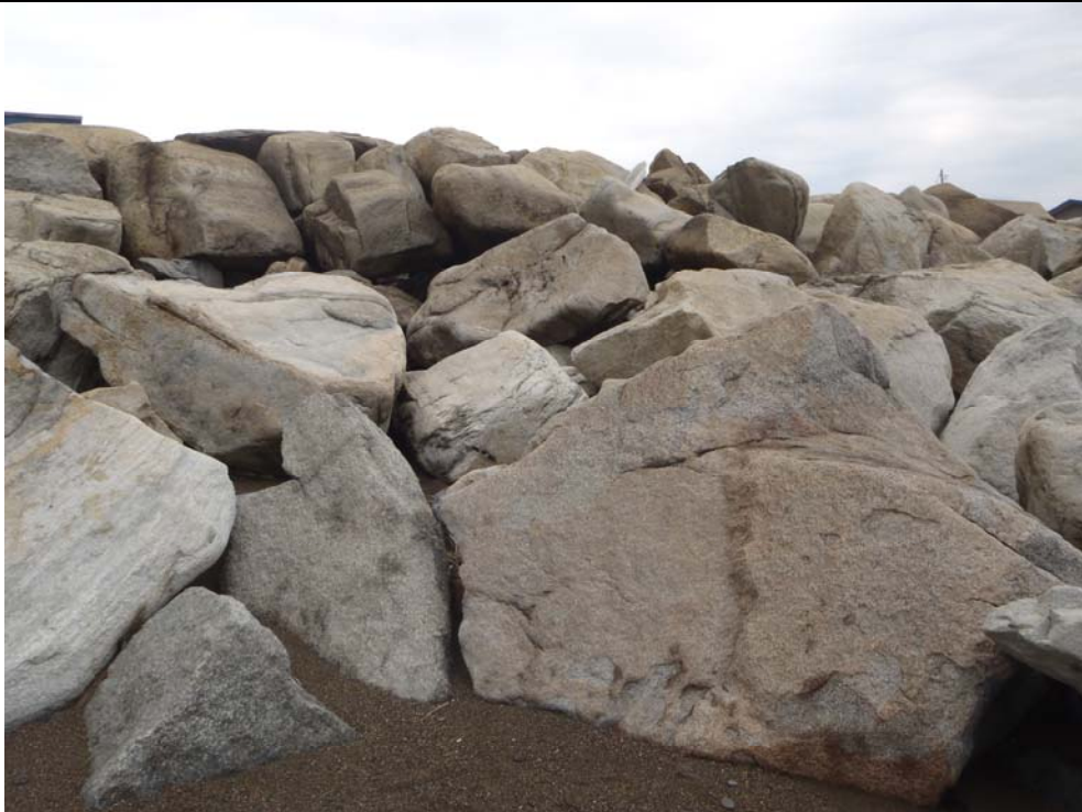
Missing armor stones near crest and at toe, rounded corners
