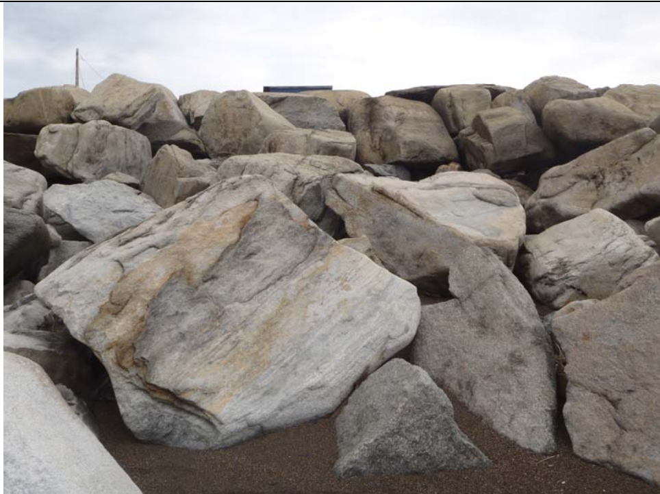
Oversteepened slope—core rock missing from 2:1 grade, rounded edges
