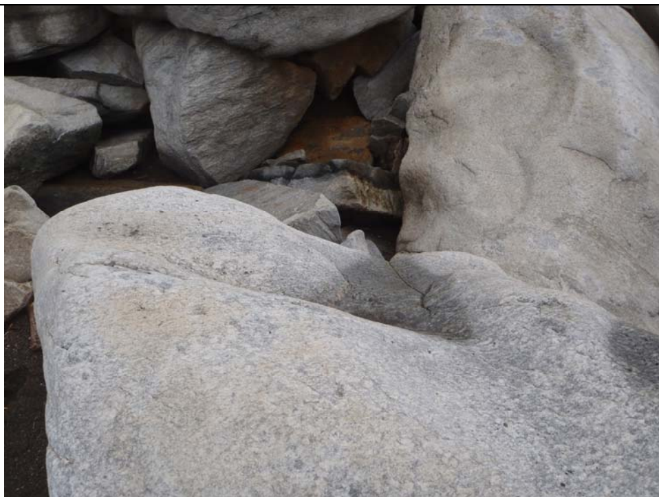
Exposed core rock, rounded edges
