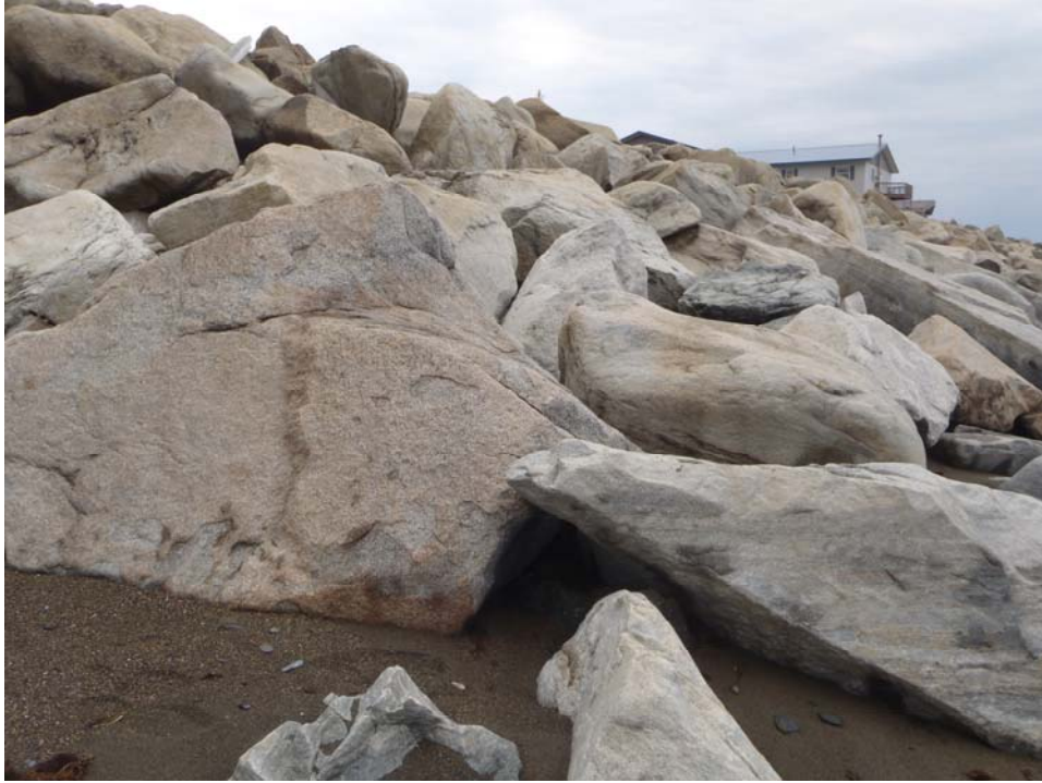
Missing toe rock, rounded corners
