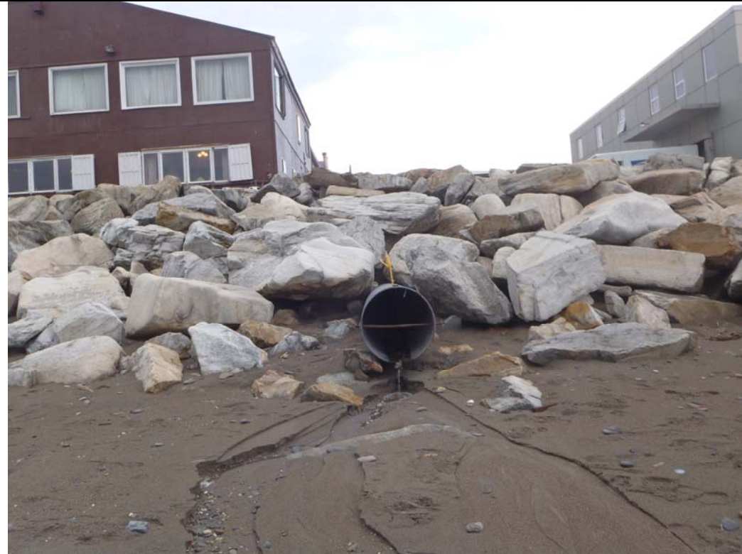
Exposed core rock at culvert
