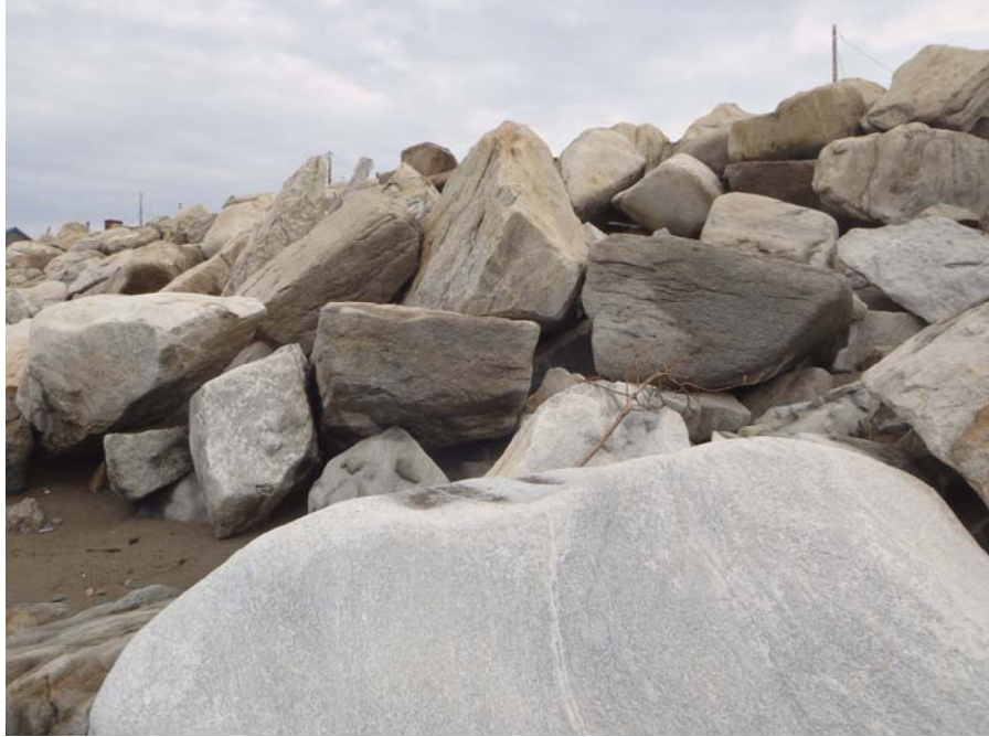
Missing core rock on 2:1 constructed slope, missing toe stones, rounded stone in foreground
