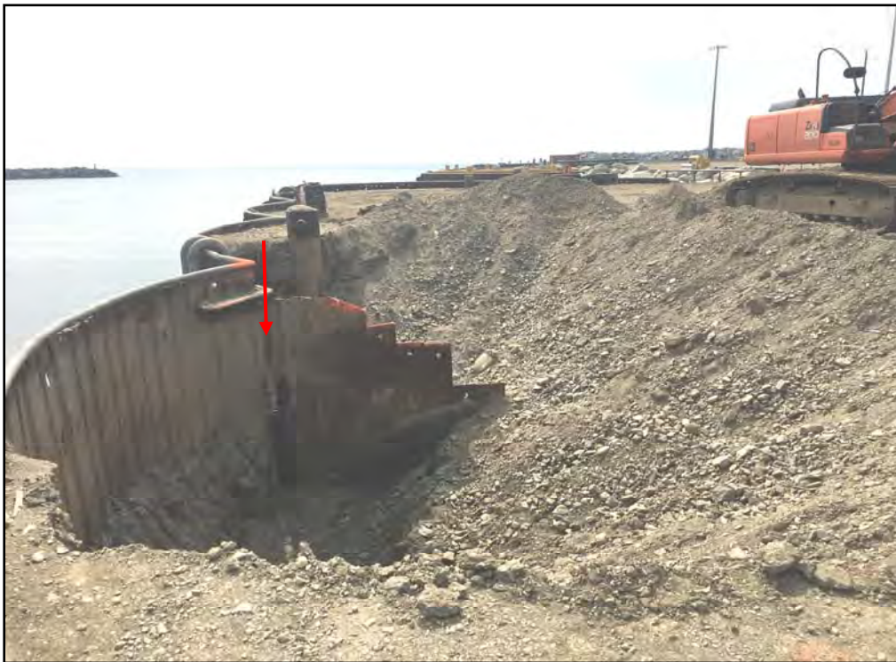
Photo 2 – West Gold Dock inside view of cracked wye joining Cells 5 and 6
