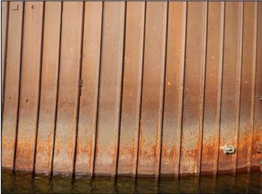
Photo 9 – West Gold Dock typical pitting corrosion at splash zone
