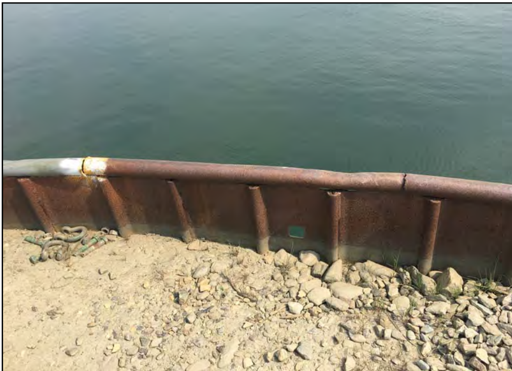
Photo 10 – West Gold Dock typical cracking on bull rail
