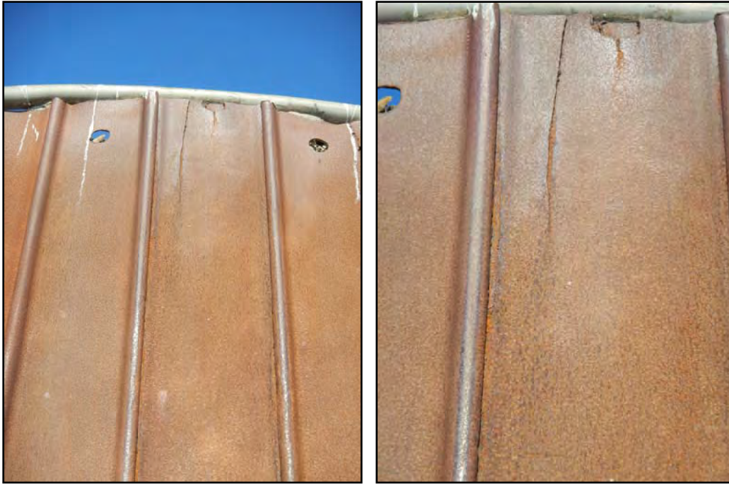
Photo 5 – West Gold Dock 2.5-foot vertical crack on Cell 4, eight sheets from Wye 4-5
