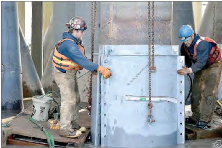
A protective jacket is installed on a wharf pile. JIM JAGER/PORT OF ALASKA
