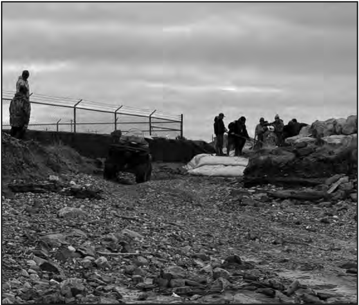
Photo courtesy Donna Barr SHISHMAREF — Shishmaref residents prepared for the weekend storm by filling sand bags for protection around the sewage and washeteria lagoons.
