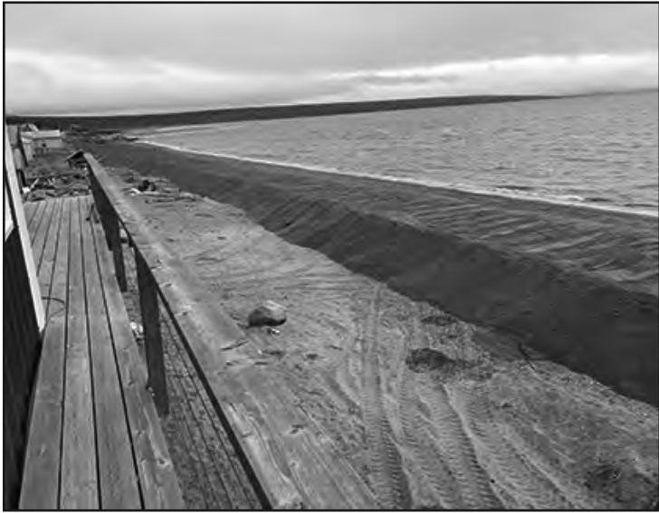
BERM — The community of Golovin built up a berm to protect houses from the wind and waves.
