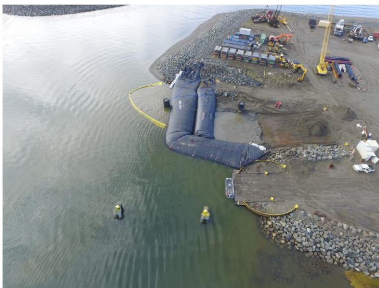
(STG AquaDam installed around the Launch Ramp Replacement Project)
