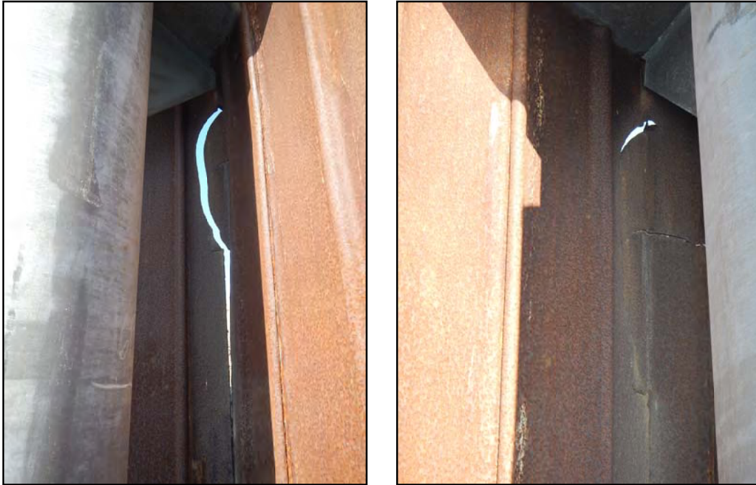
Photo 3 – West Gold Dock outside views of cracked wye joining Cells 5 and 6
