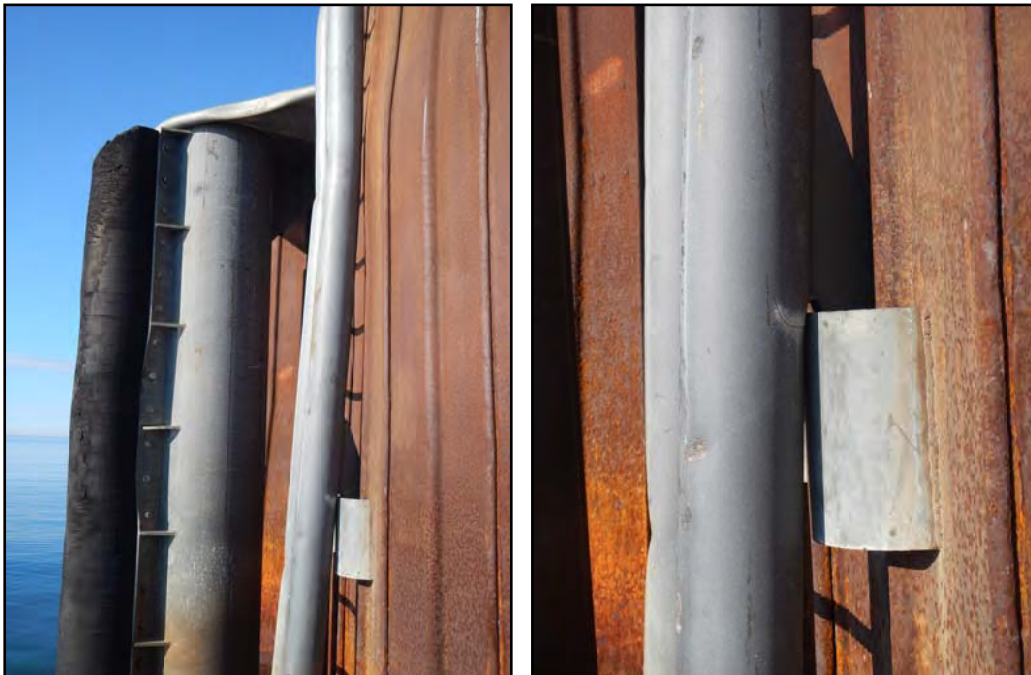
Photo 6 – West Gold Dock cracked and bent ladder at Wye 3-4
