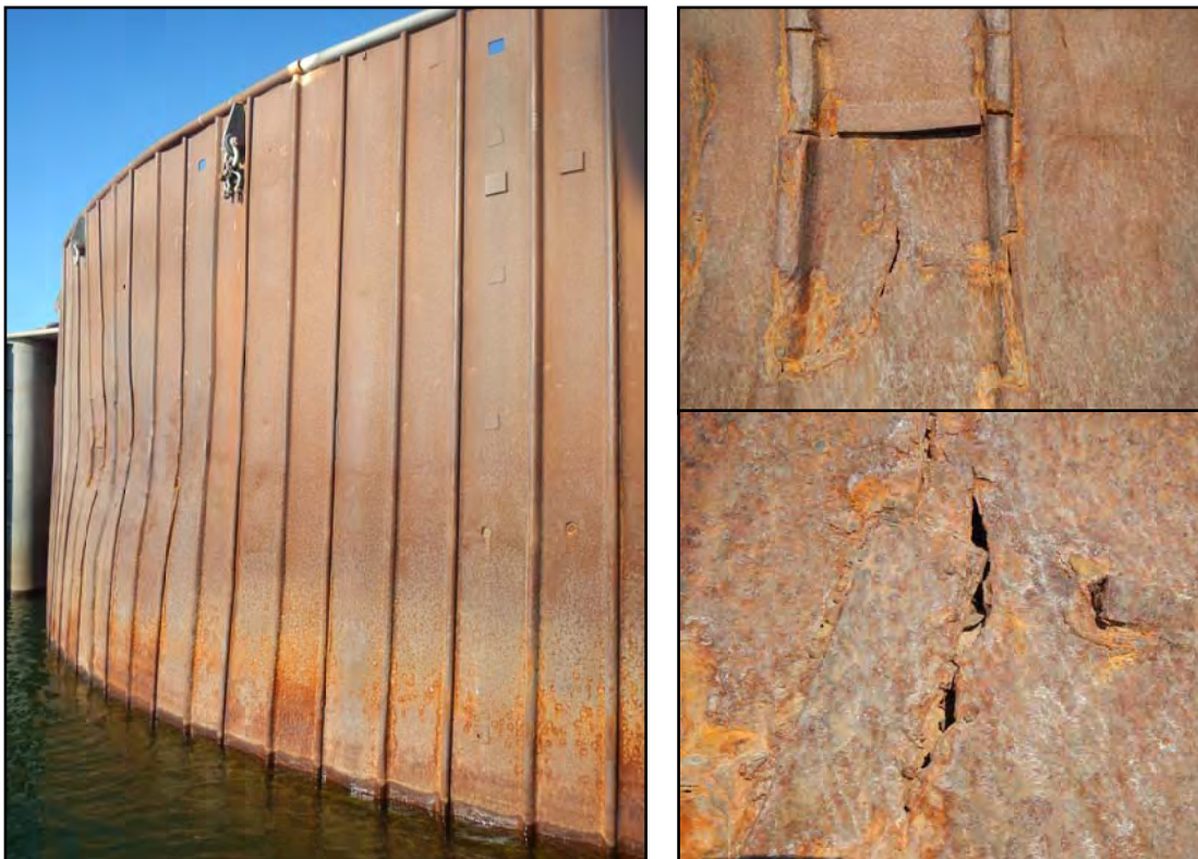
Photo 4 – West Gold Dock large dent and cracking on Cell 8
