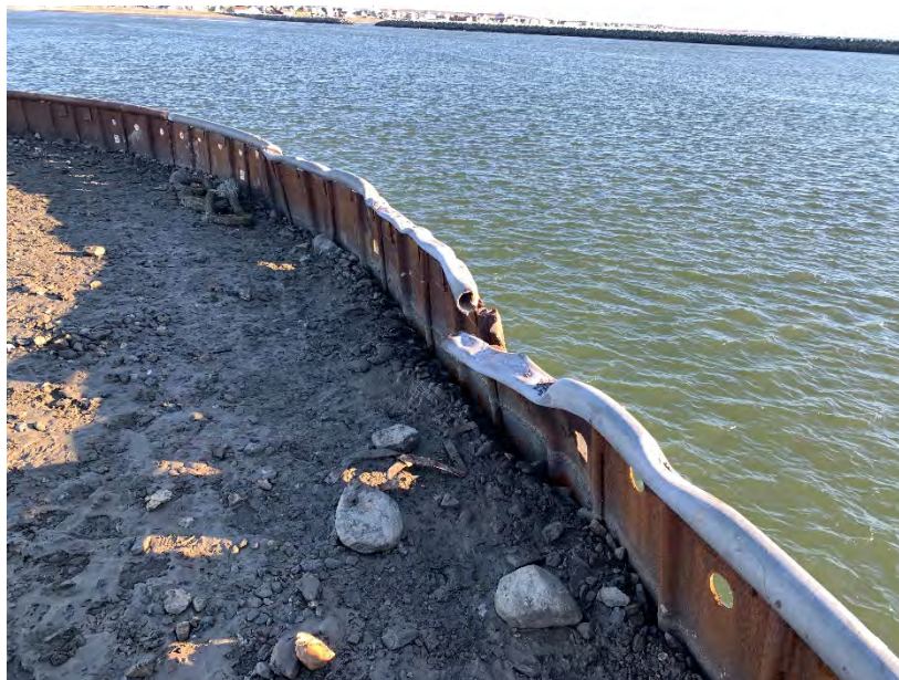
Figure 9: West Gold Dock cell damage
