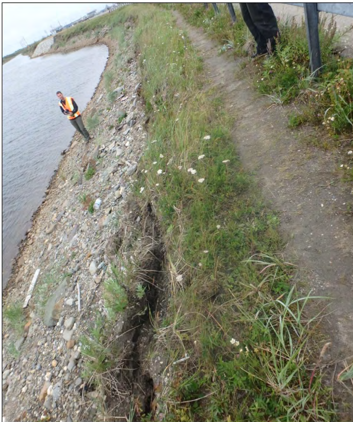
Figure 2. Tension crack at top of Snake River bank, upstream of new bridge. PDC Engineers photo.
