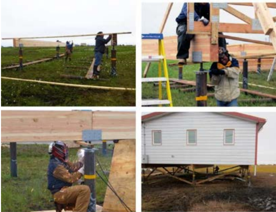
Figure 26. Example use of Saddle Bracket jacks over piles to adjust elevation due to soil settlement resulting from thawing effect in active layer and permafrost zone (CCHRC 2014)
