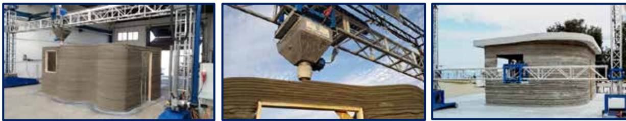
Figure 21: Images and Summary of BeMore3D Printer Characteristics
