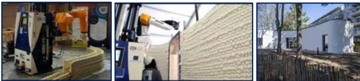
Figure 20: Images and Summary of Batiprint3D Printer Characteristics
