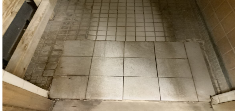
Worn Out from Heavy Usage: The women's sauna is in particularly poor condition. Years of neglect have led to loss of grout and rotten subflooring. Floor has hard water stains throughout.
