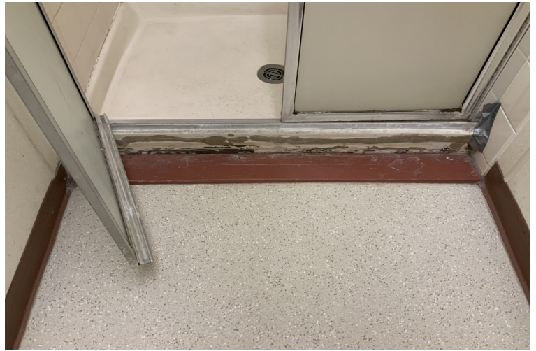
Rotten Flooring and Sub-Flooring: Water has been escaping the shower pan in one of the single showers in the ladies' locker room leading to rotten flooring and unsafe conditions.
