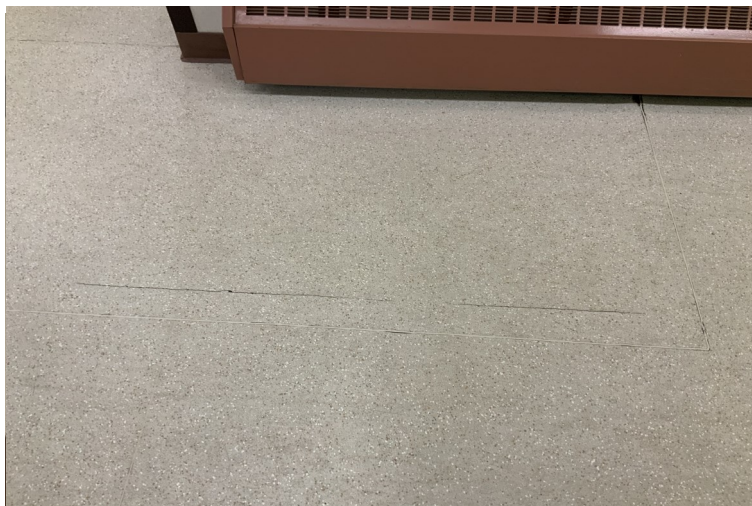
Old Worn Flooring: Heavy traffic and repeated use have lead to cracks forming on the floor of the women's locker room. As the degradation continues water will seep down into the subfloor.
