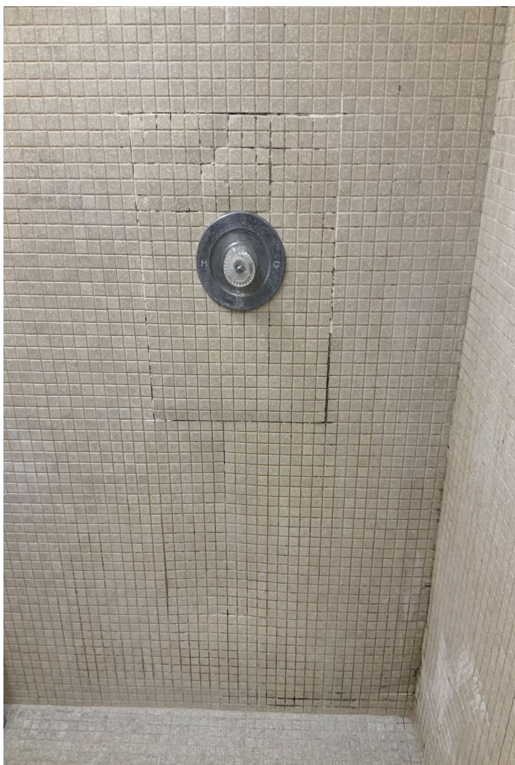
Needs Immediate Attention: Water has permeated the tile in the women's group shower so thoroughly that the walls are collapsing as evidenced by the wavy pattern visible above. In the lower right corner it is completely rotted.
