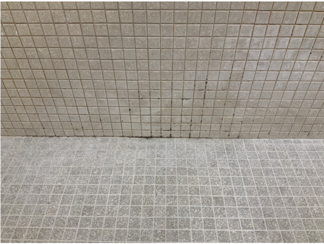
Mold in Grout of Men's Showers: Once mold gets into grout it is impossible to remove. Staff have tried numerous ways to remove it and none have been successful.
