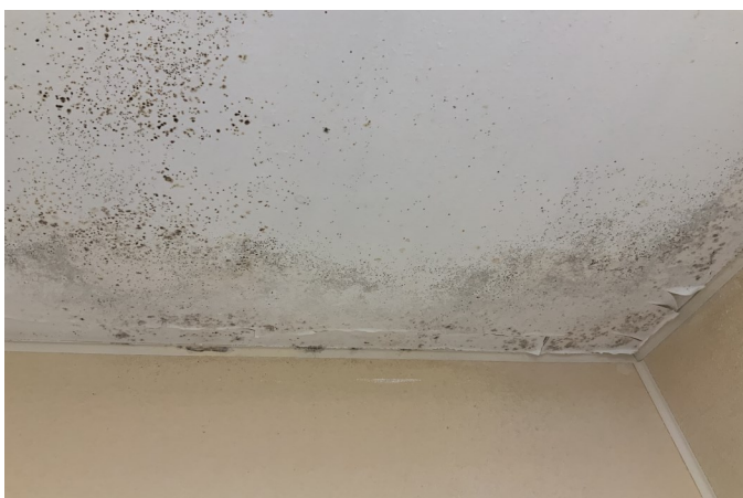
More Mold in the ceilings: The existence of mold is pervasive throughout the ceiling areas of both locker room ceilings.
