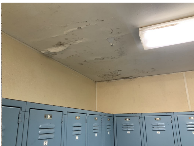
Mold Growing on the Ceiling: Lack of ventilation has led to mold growth on the ceiling of the men's locker room. The build-up of moisture is making the plaster peel.
