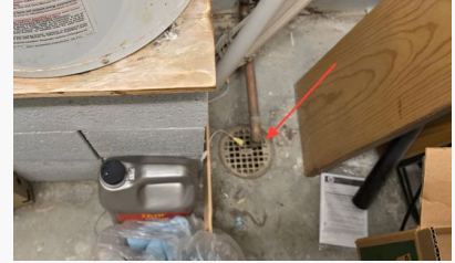
floor drain in storage/utility room
