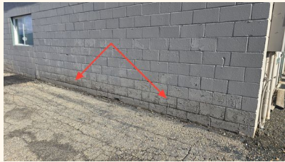
failing paint
